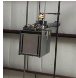
Gas-Fired Unit Heater and Programmable Thermostat
