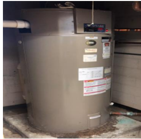
Condensing Water Heater
