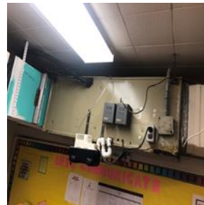
Indoor Fan Coil Unit & Programmable Thermostats
