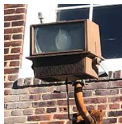
Exterior Fixtures (Metal Halide & CFL)
