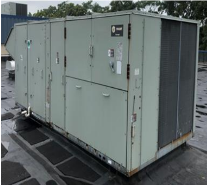
Large Trane Package (RTU)
