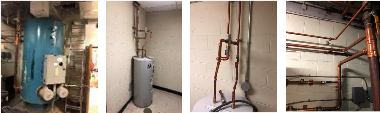
Electric Domestic Hot Water & Uninsulated Pipes
