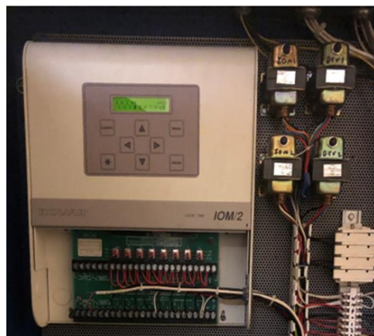
Hot Pumps & Novar Control System
