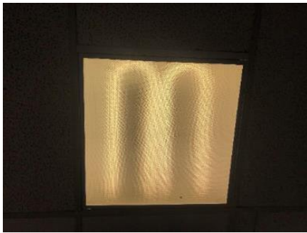
U-Shape 2-Foot T8 fixture
