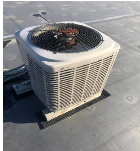
Packaged Terminal Heat Pump & Split System AC
