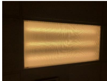
Linear 4-foot T8 fixture
