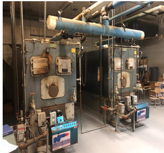
Newer & Older Sections Hot Water Boilers
