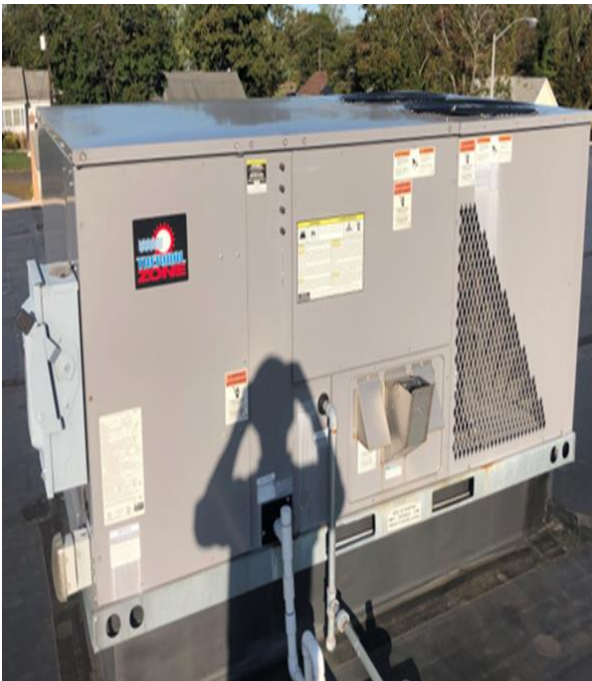
Thermal Zone Packaged Unit
