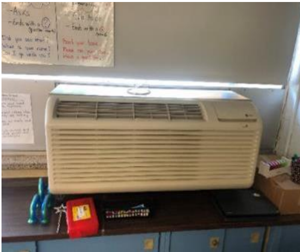
Packaged Terminal Heat Pump & Split System AC
