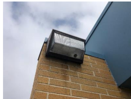
Exterior wall pack fixture
