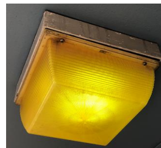
Exterior HPS Recessed Fixture
