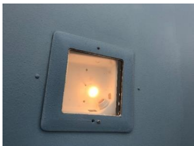
Exterior Recessed Incandescent fixture
