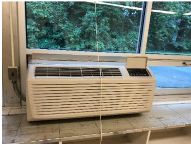
Packaged terminal heat pumps
