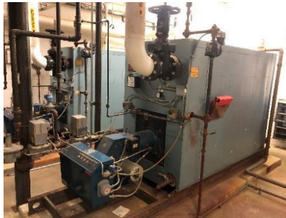
Non-condensing hot water boilers
