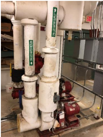
Chilled water pump insulation
