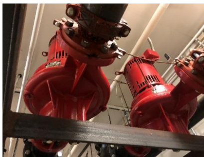
Heating hot water pumps
