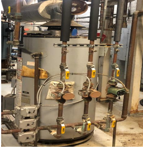
DHW & Insulated Hot Water Pipes
