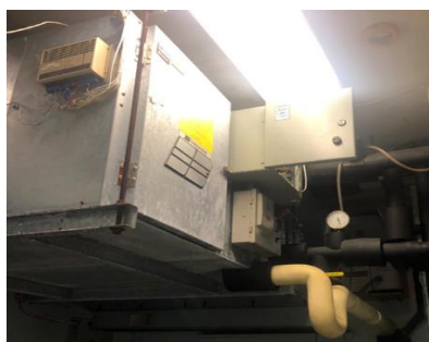
Air Handling Unit (AHU) & Novar Control System
