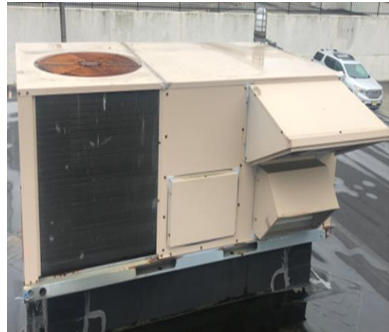
Unit Ventilator & York Packaged Air Source Heat Pump
