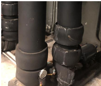
Dual Temperature 7.5 HP Hot Water Pumps
