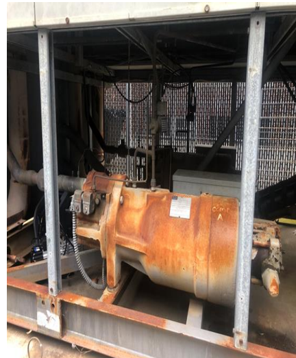
Trane Air Cooled Screw Chillers & Compressor
