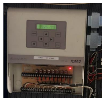
Air Handling Unit (AHU) & Novar Control System
