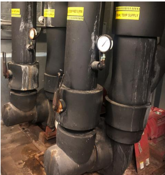
Dual Temperature Chilled Water Pumps
