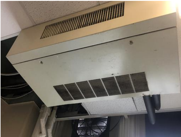
Unit Ventilator & York Packaged Air Source Heat Pump
