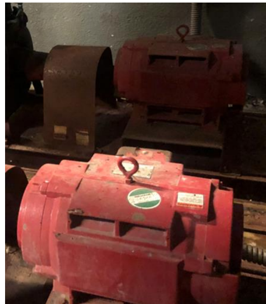
Dual Temperature Chilled Water Pumps
