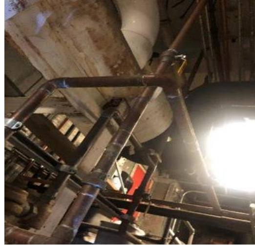
DHW & Insulated Hot Water Pipes
