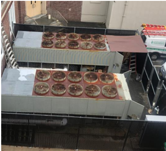
Trane Air Cooled Screw Chillers & Compressor
