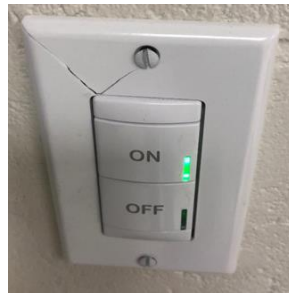
Wall Mounted Occupancy Sensor
