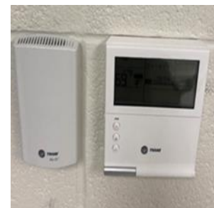
Programmable Thermostats
