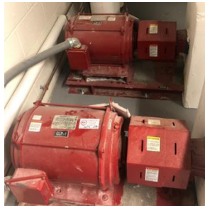
Heating Water Circulating Pumps
