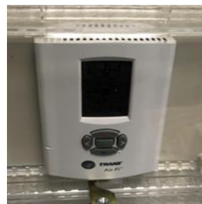
Programmable Thermostats
