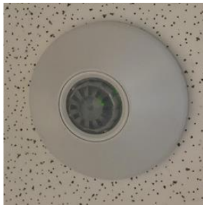
Ceiling Mounted Occupancy Sensor
