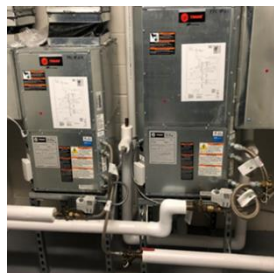
Water Source Heat Pumps
