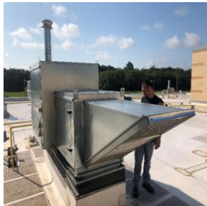
Make Up Air Unit (MUA)
