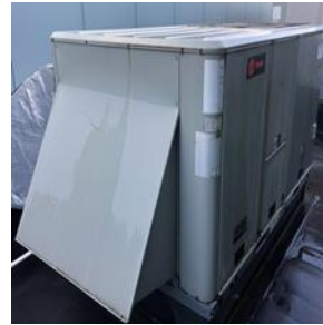
Packaged Heat Pump Unit
