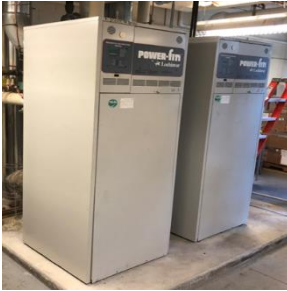
Condensing Boilers
