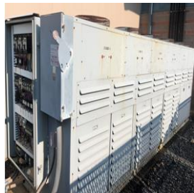
Central Kitchen Walk-ins Condensing Unit
