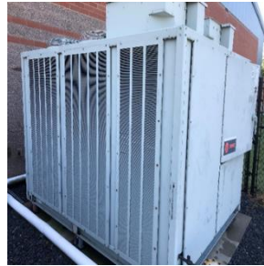
Trane AC Condensing Unit
