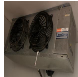
Walk-in Unit Evaporator
