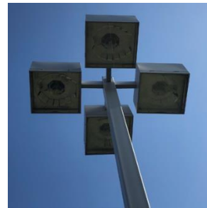
HID Pole Mounted Fixture
