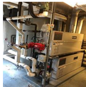
Newer Wing Domestic Hot Water System
