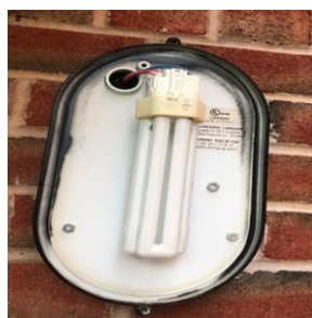
CFL in Porch Wall Mounted Fixture
