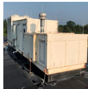
Trane Air-Cooled Condensing Unit & Attached Gas-fired Furnace
