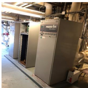
New Wing Condensing Boilers, Hot Water Pumps & Hot Water Control Loop
