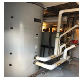
Newer Wing Domestic Hot Water System
