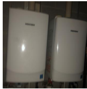
Tankless Gas-Fired Water Heaters
