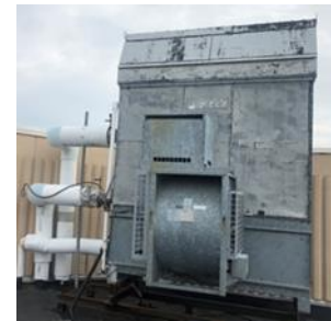
WSHP Heat Rejection Cooling Tower
