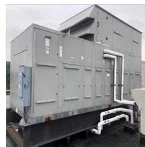
Pool Dehumidification Unit
