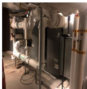
Indoor Carrier AHU
