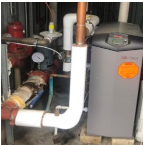
Condensing Boiler
