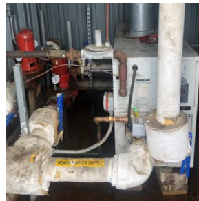
Non-Condensing Boiler
