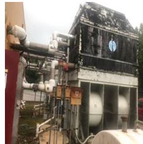
Three One-Cell Cooling Tower
