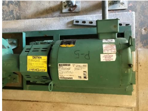
Heating hot water pumps
