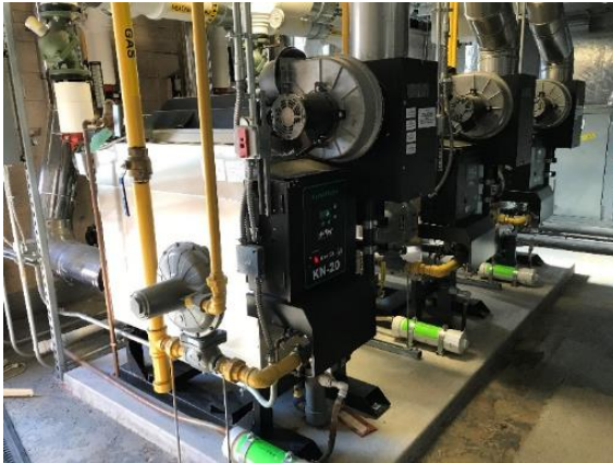
Condensing boilers
