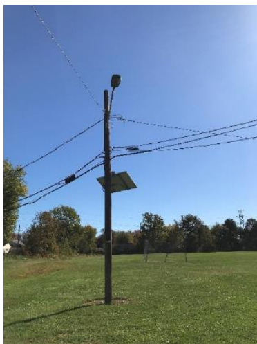
Pole fixture – High Pressure Sodium
