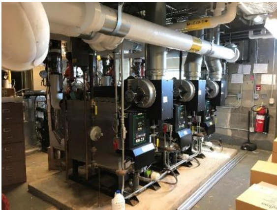
Condensing boilers
