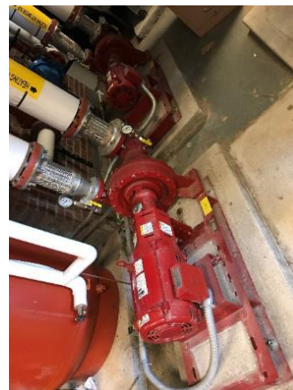
Heating hot water pumps
