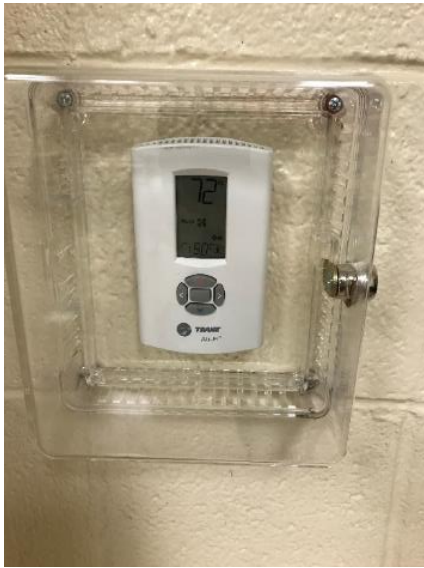
Programmable Thermostat
