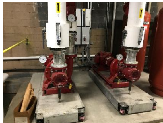
Heating hot water pumps
