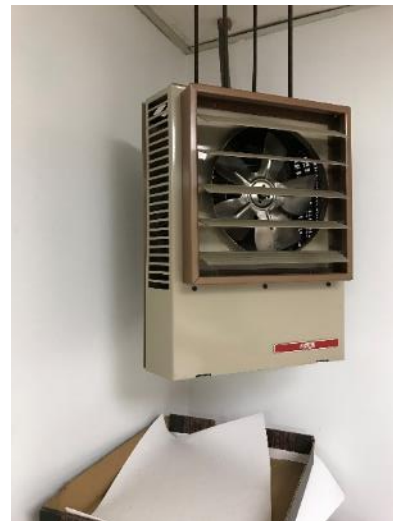
Electric Unit Heater
