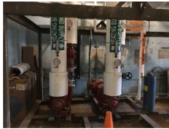
Heating hot water pumps
