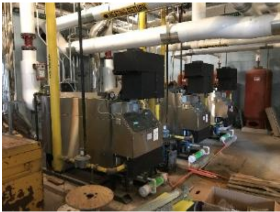
Condensing boilers
