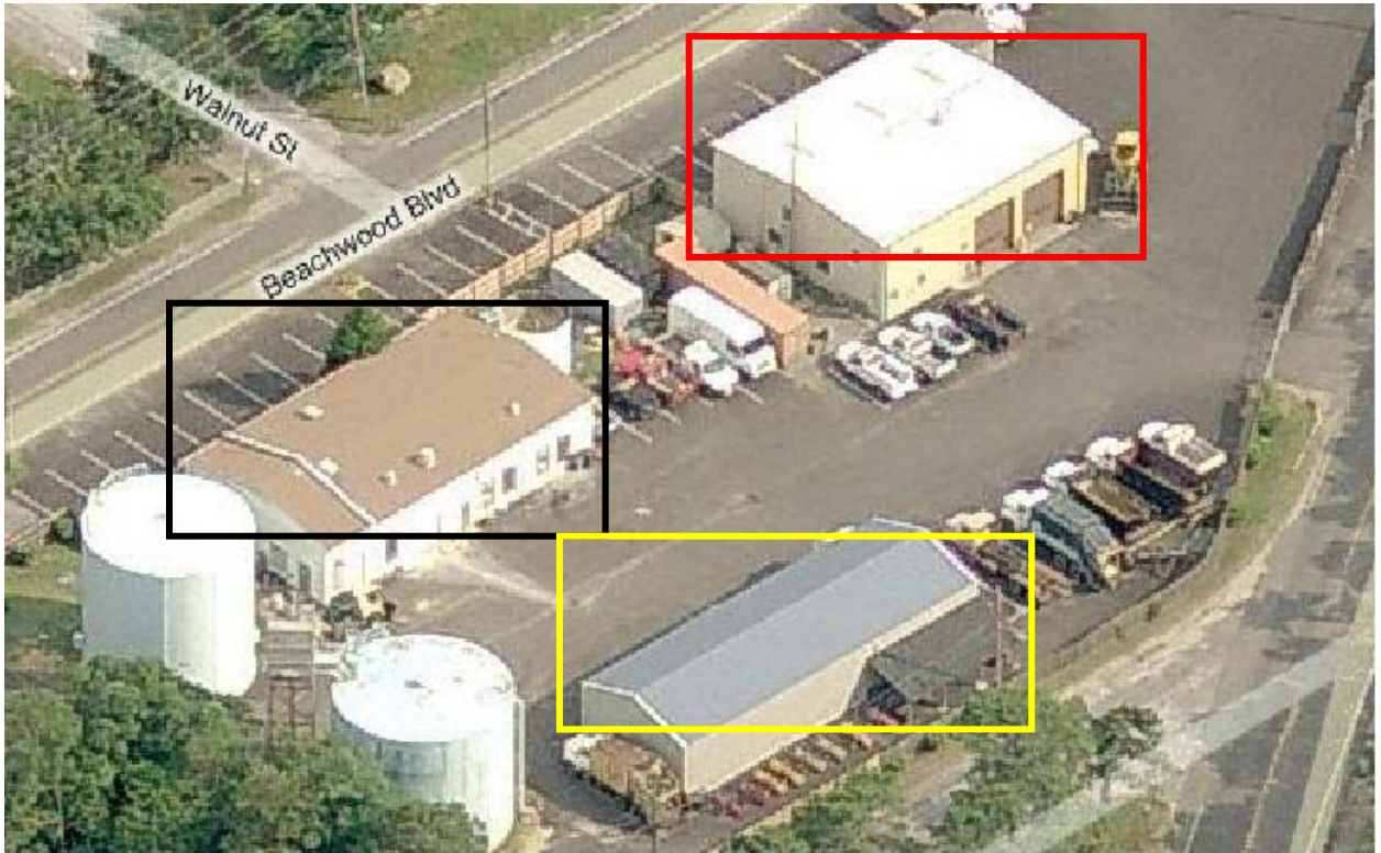
Outlined in Red in the above image is DPW Garage steel roof. Outlined in Black above is the Water Dept. building asphalt shingled roof. Outlined in Yellow in the above image is a three walled steel structure used to store vehicles.
