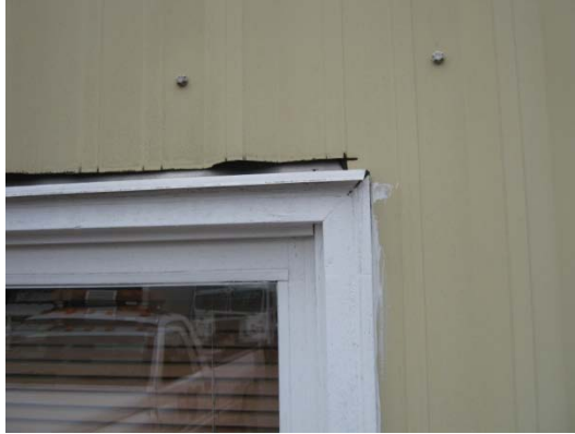
Single Pane Aluminum Window on the Garage
