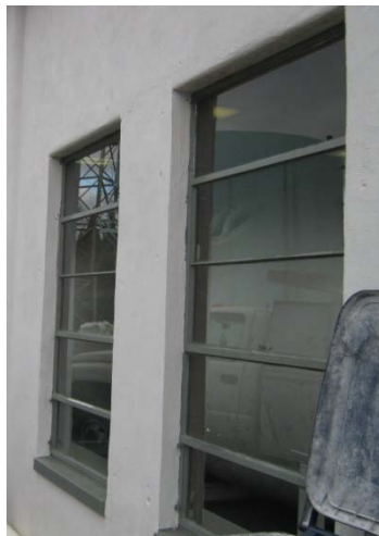
Single Pane Aluminum Window on the Water Dept building
