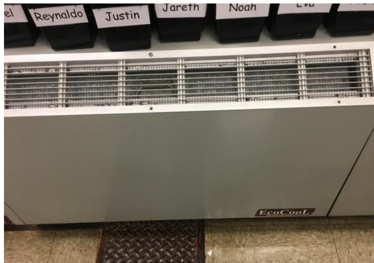
Picture 5: Sample Horizontal Heat Pump
