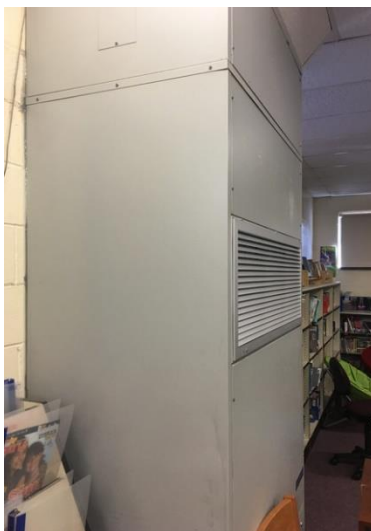
Picture 4: Sample Vertical Heat Pump
