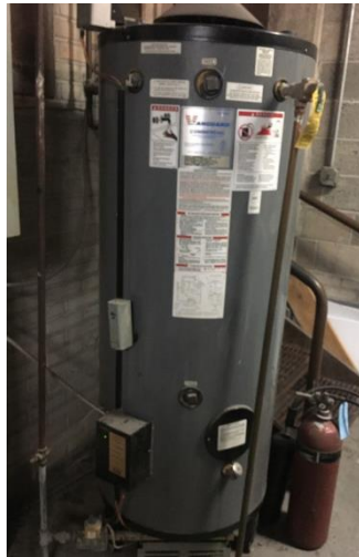
Picture 6: Existing Natural Gas Heater
