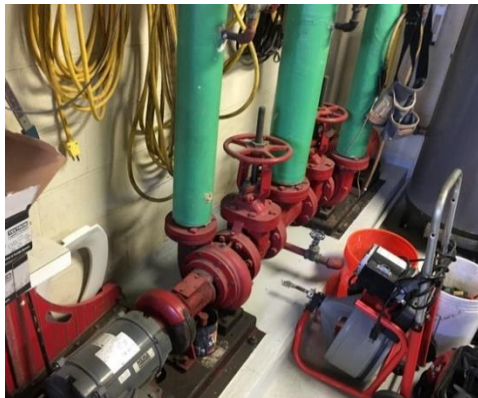
Picture 8: HW Supply Pumps
