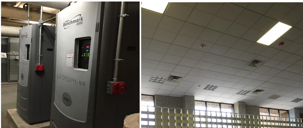
Image 3 Boilers and terminal units
