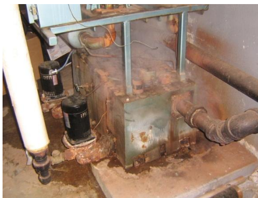
Condensate Receiver Pump Set with Rusted Body, Leaking Steam
