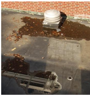
Signs of pooling, drain issues and cracked built-up roofing seams found
