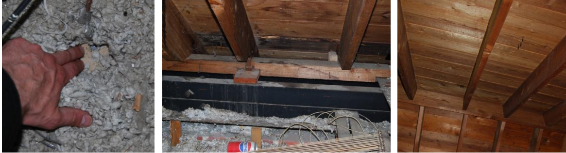
Insufficient ceiling insulation and no-existent attic ventilation in the original building sections
