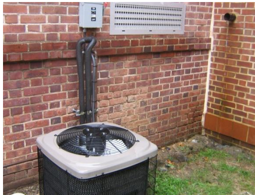
Typical Condensing Unit Piped to Classroom Unit Ventilator
