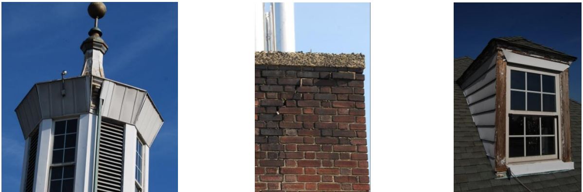
Center cupola, chimney and some dormers in need of repair
