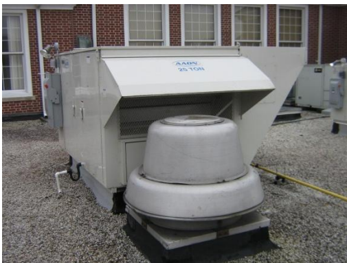
Exhaust Fan Located Beneath Aeon Out-side Air Intake Hood
