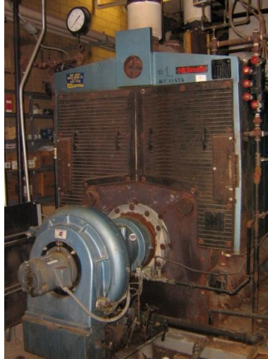
One of the Three Steam Boilers in the North Boiler Room
