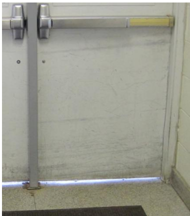
Signs of worn or missing weather stripping at doors and roof hatch
