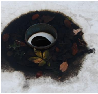
Signs of pooling, drain issues and cracked built-up roofing seams found
