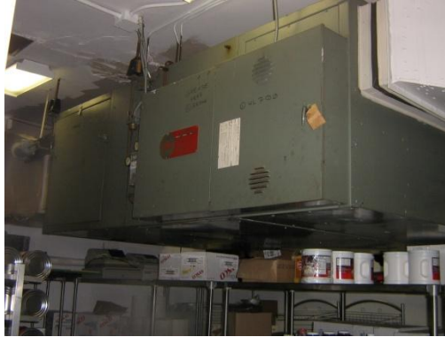
Original Steam H&V Unit Serving the Kitchen
