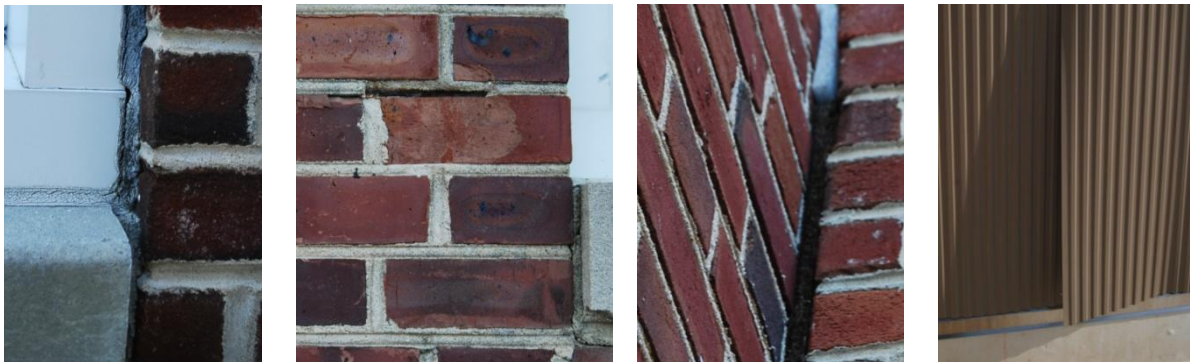
Cracked caulk, bricks and mortar and loose parapet metal wall panels were found
