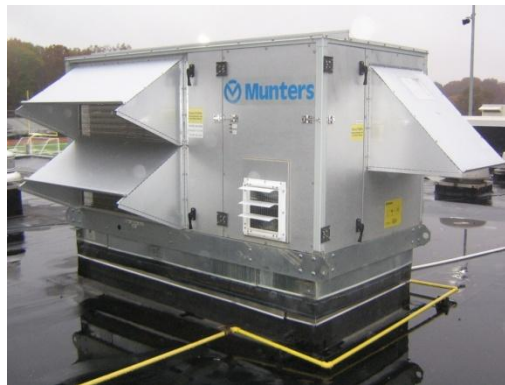
Energy Recovery Unit Serving the Gym Area
