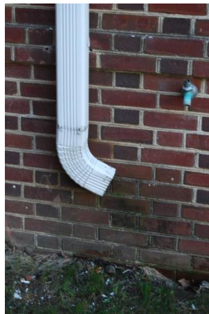
Ineffective downspout / discharge directions in various locations
