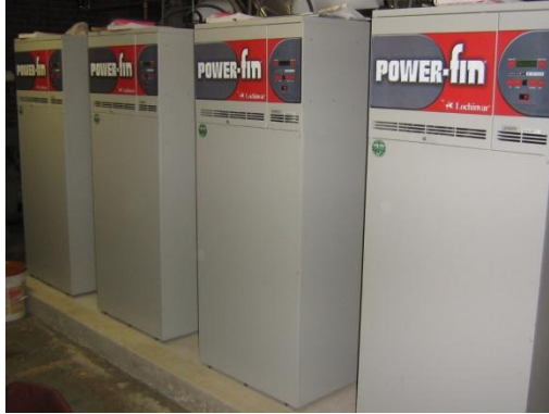
Hot Water Boilers In South Boiler Room
