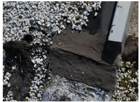
Signs of pooling, drain issues and cracked built-up roofing seams found
