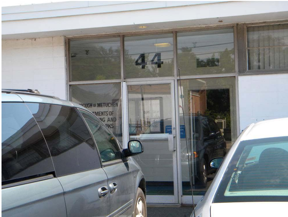
The glass is new on the entry and doors but there is no weather-stripping at all.
