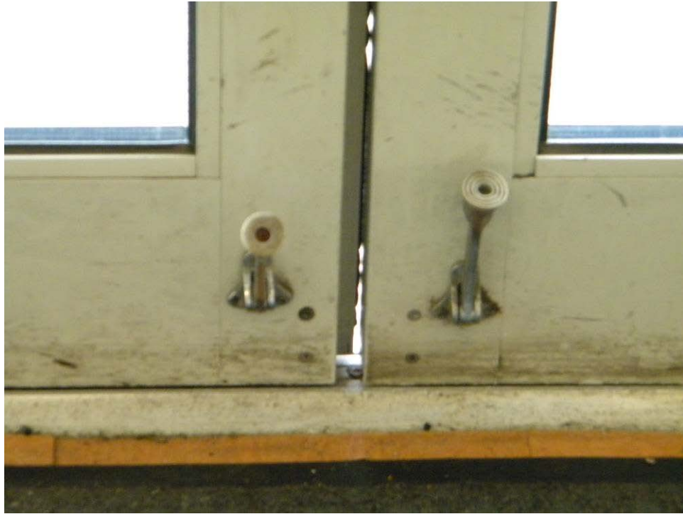
Daylight can be seen between the two main entry doors
