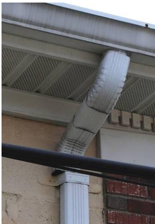
Dislocated, Clogged and Missing Down-Spouts at Side Walls
