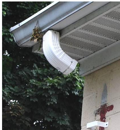
Dislocated, Clogged and Missing Down-Spouts at Side Walls
