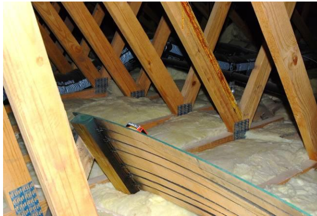
Existing Attic Insulation Conditions
