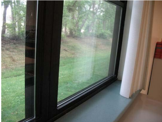
Double Pane Windows in good condition
