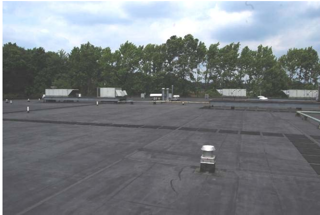
EPDM rubber membrane roofing in fair condition
