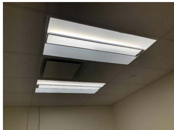
LED Direct/Indirect Fixtures
