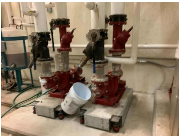
Heating Hot Water Pumps
