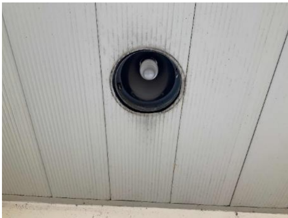
Recessed Can Fixture – Metal Halide
