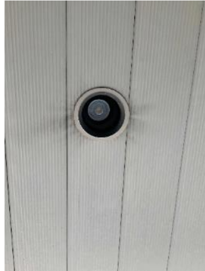
Recessed Can Fixture - LED
