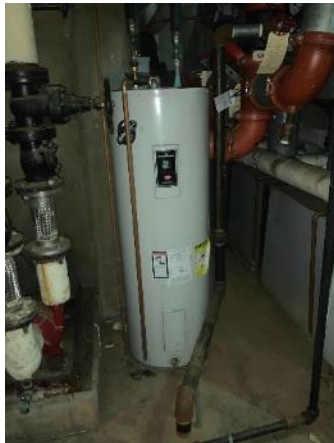
Electric DHW Tank - Main
