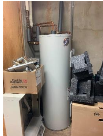
Electric DHW Tank - Storage
