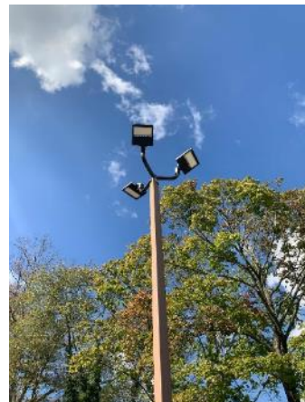
Triple Head Pole-Mounted Fixture
