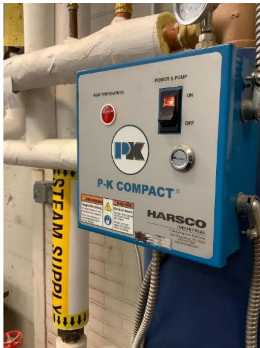
DHW Heat Exchanger Control
