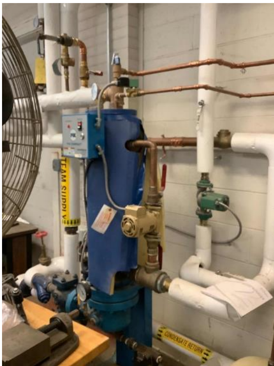
DHW Heat Exchanger
