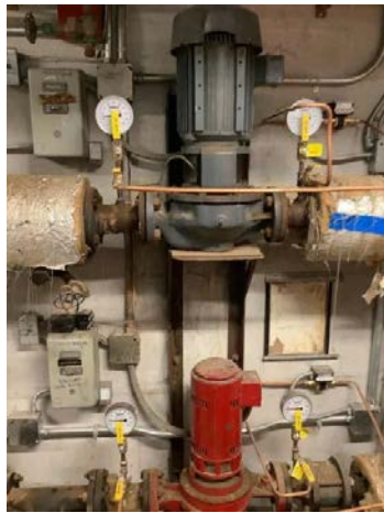
Heating Hot Water Pumps
