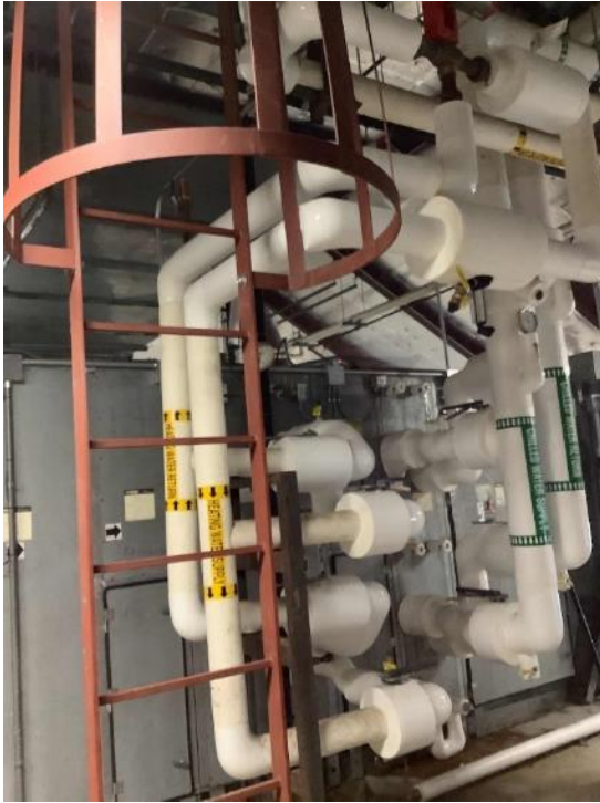
AHU HW & CHW Piping
