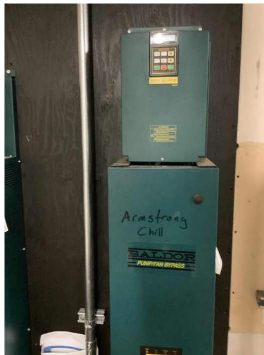
Chilled Water Pump Control
