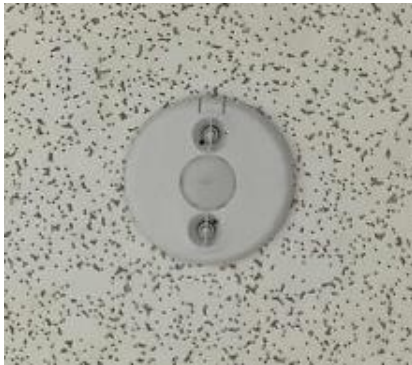
Ceiling Mounted Occupancy Sensor
