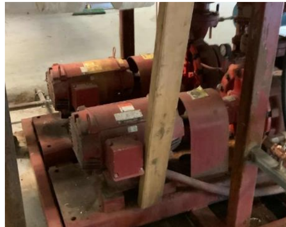
Heating Hot Water Pumps
