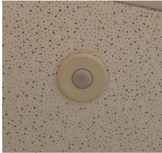
Ceiling Mounted Occupancy Sensor
