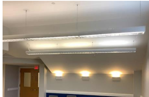
Pendant Mounted & Wall Wash Fixtures
