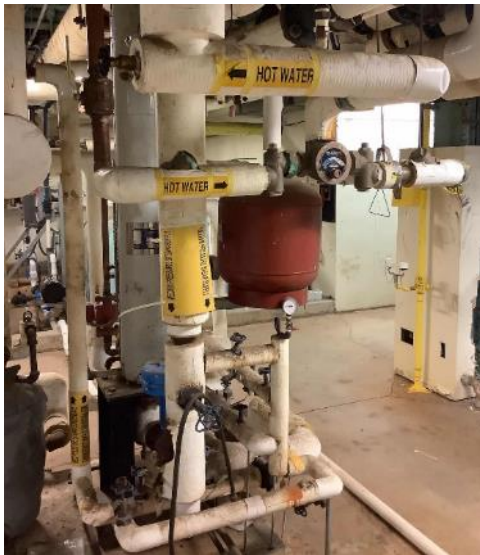
Heating Heat Exchanger
