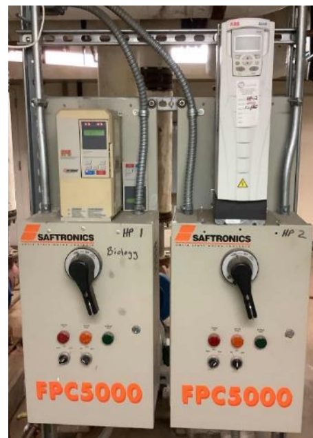
Hot Water Pump Controls
