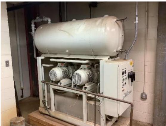
Medical Air Pump Air Compressor
