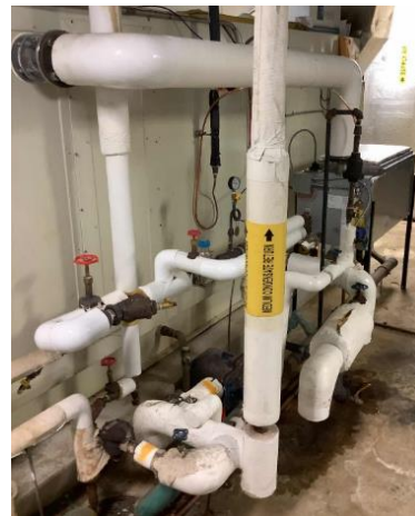
AHU-5 Steam Humidifier System
