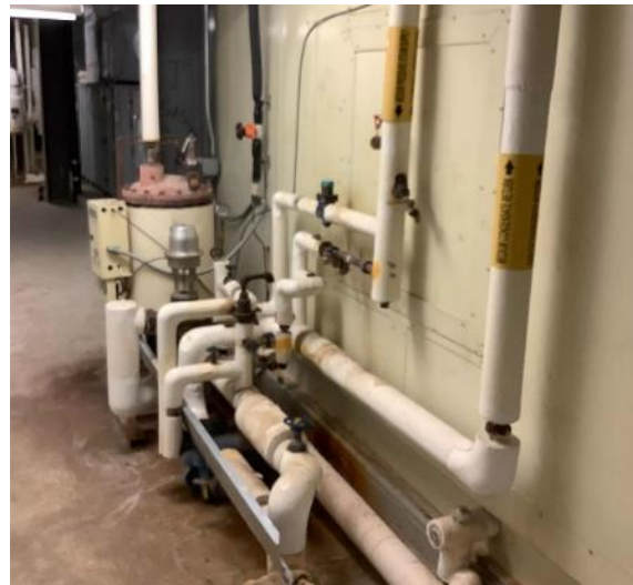
DHW Heat Exchanger
