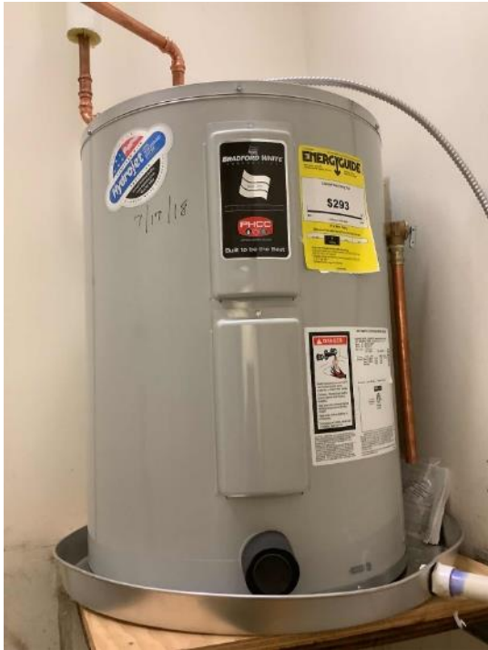
Bliss Annex DHW Storage Tank Water Heater
