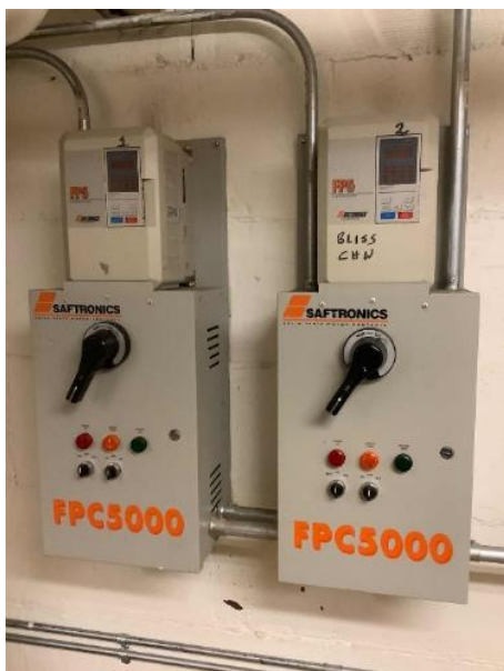
Bliss Hall Chilled Water Pump VFDs
