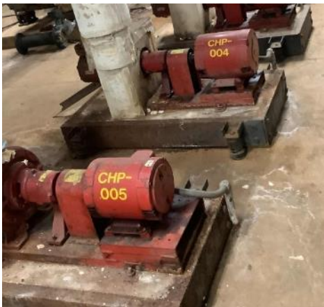
Bliss Annex Chilled Water Pumps
