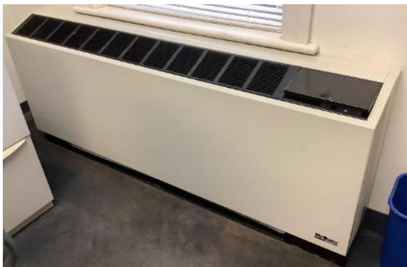
Bliss Hall Unit Ventilator
