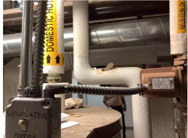
Bliss Hall DHW Circulation Pump
