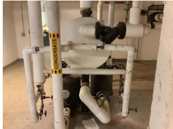
Bliss Hall Heat Exchanger
