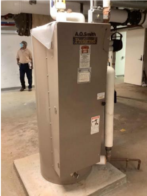
Bliss Hall DHW Storage Tank Water Heater
