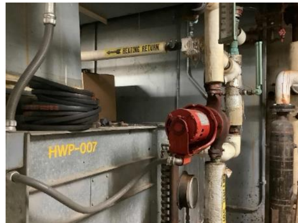
AHU-002 Hot Water Circulation Pump
