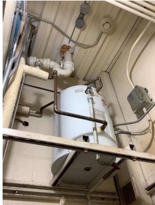
Bliss Annex DHW Storage Tank Water Heater
