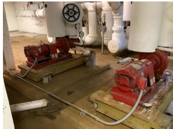
Bliss Hall Chilled Water Pumps
