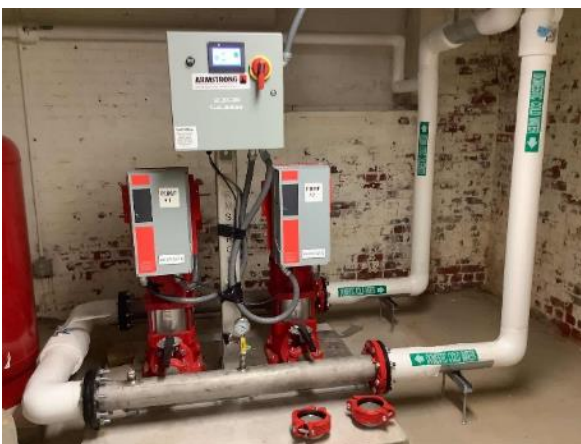
Bliss Hall Cold Water Supply Pumps
