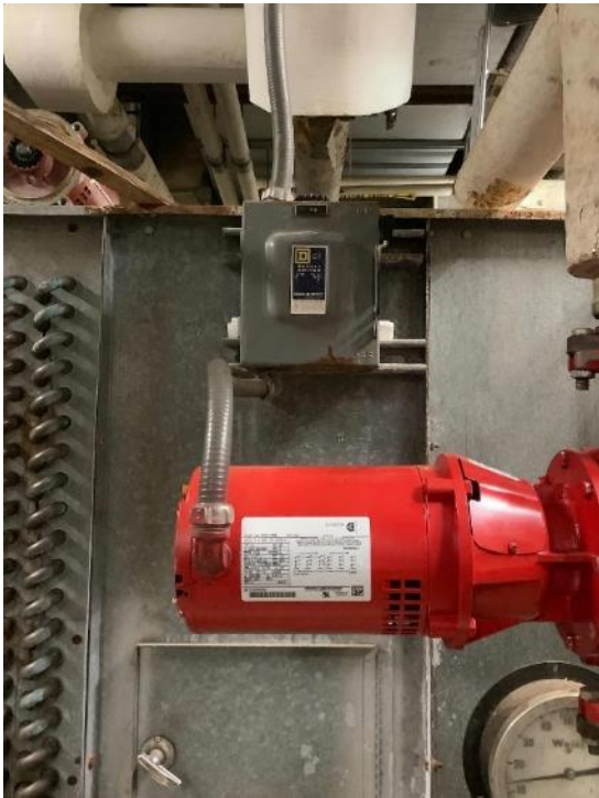
AHU-001 Hot Water Circulation Pump
