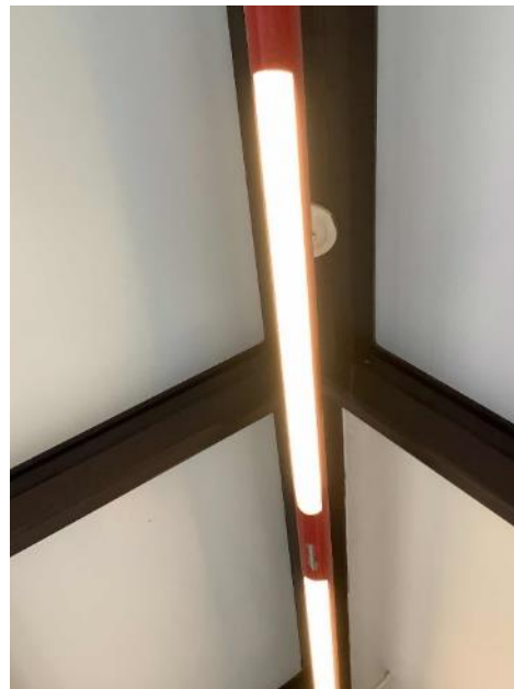
Walkway Pendent Mounted Fixtures
