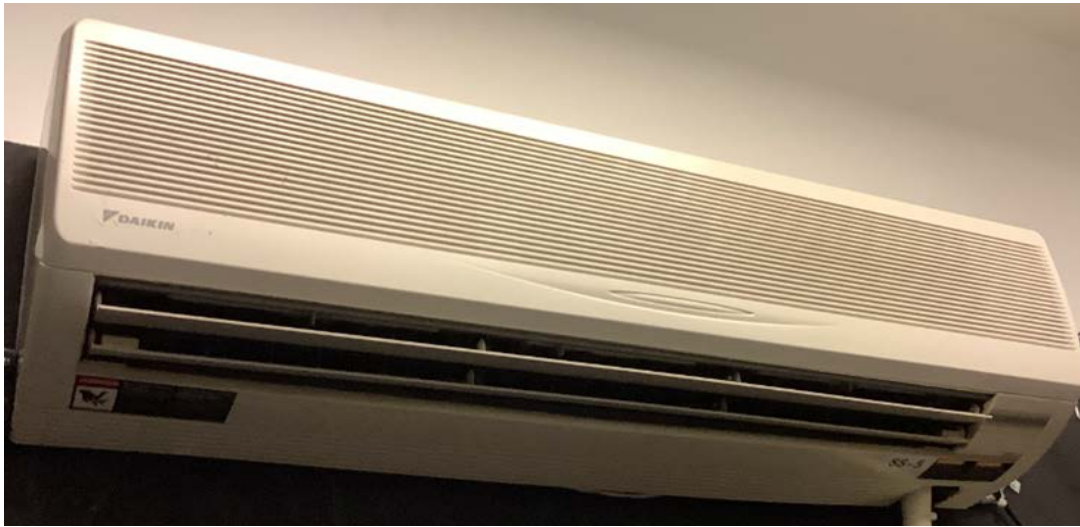
Ductless Split System Evaporator
