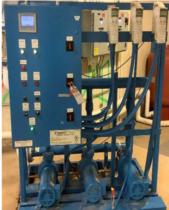
0.5 hp Domestic Hot Water Pumps & 5 hp Booster Pumps
