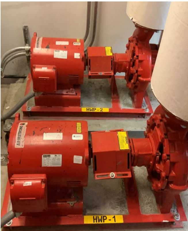
Main Hot Water Pumps & Variable Frequency Drives (VFDs)
