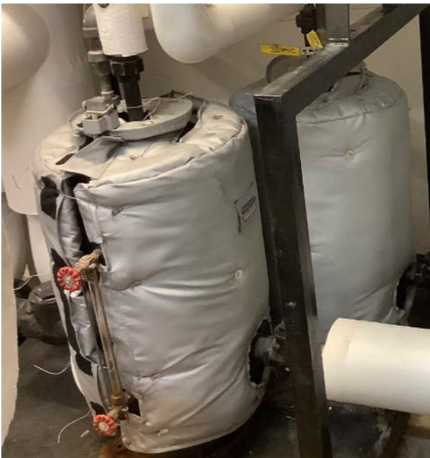
Pressure Induced & 3 hp Condensate Pumps
