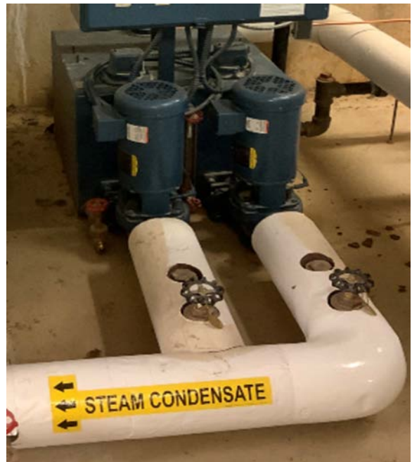
Pressure Induced & 3 hp Condensate Pumps
