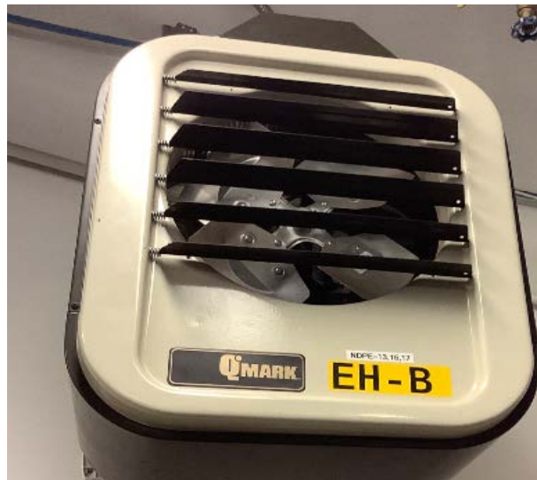
Electric Resistance Heater
