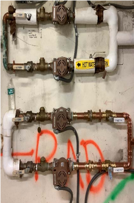
0.5 hp Domestic Hot Water Pumps & 5 hp Booster Pumps
