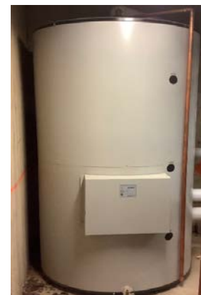
Indirect Fired Semi-Instantaneous Water Heater & Storage Tank
