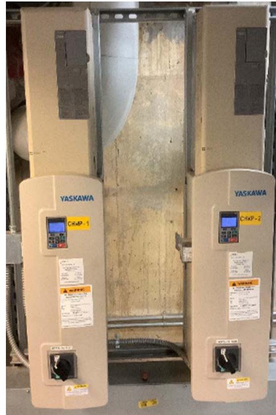
Chilled Water Pumps & VFDs
