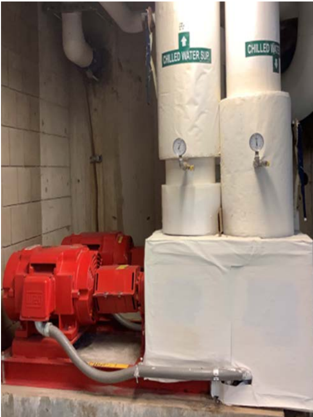
Chilled Water Pumps & VFDs
