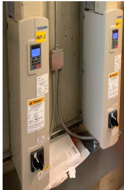
Main Hot Water Pumps & Variable Frequency Drives (VFDs)
