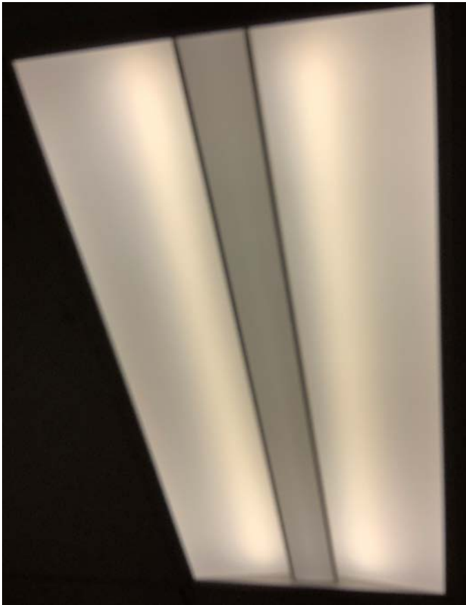
LED Fixture & Linear Fluorescent Troffer
