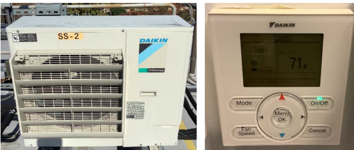
Ductless Split System Condensing Unit & Programmable Thermostat
