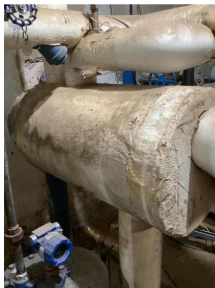
DHW Heat Exchanger
