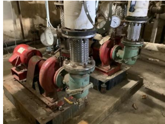
Heating Hot Water Pumps
