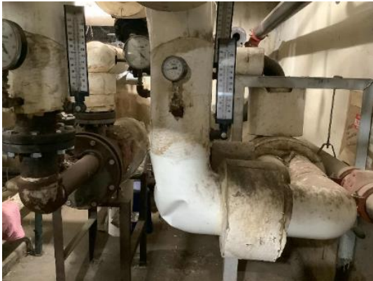
Steam Heat Exchanger System
