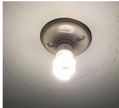
Ceiling Mounted CFL Fixture
