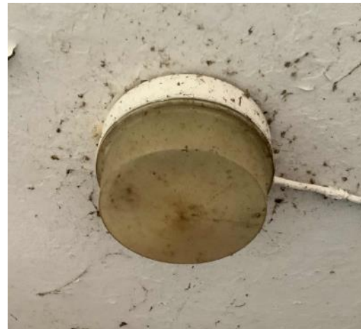
Under Canopy Mounted Fixture
