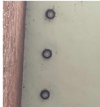
Under Canopy Recessed Can Fixtures
