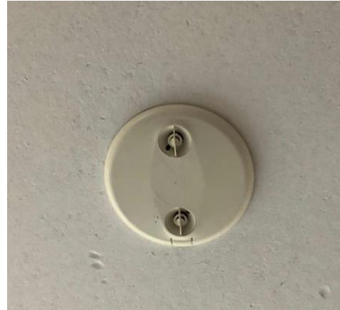
Ceiling Mounted Occupancy Sensor
