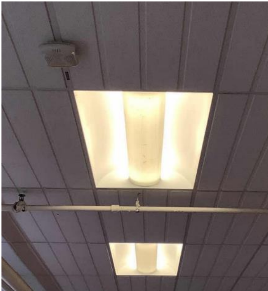
Direct/Indirect Fixtures
