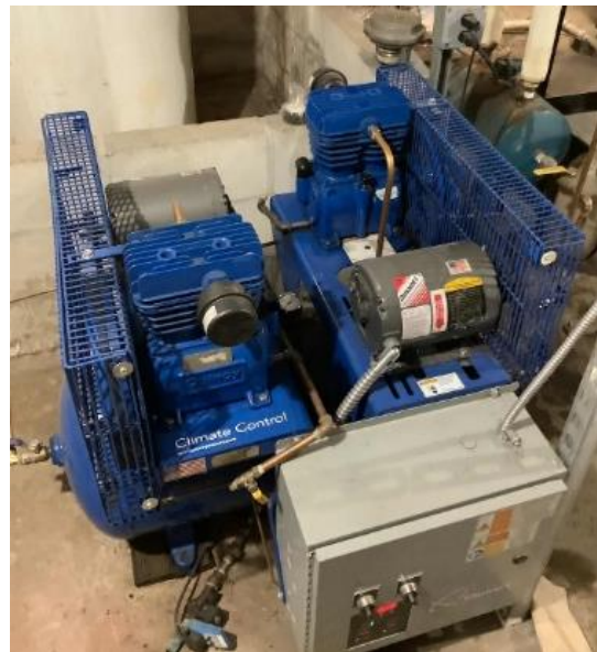
Air Compressor for Pneumatic Controls
