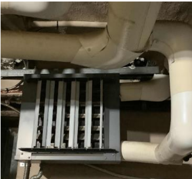
Mechanical Room Radiant Heater
