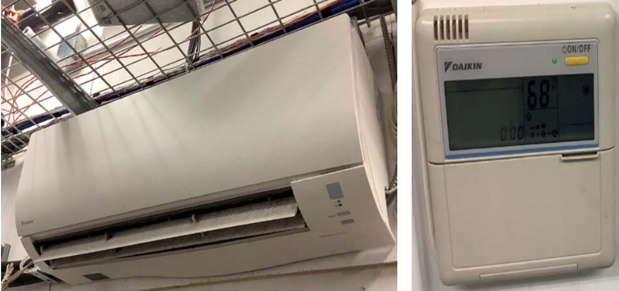
Daikin Ductless Split AC & Programmable Thermostat
