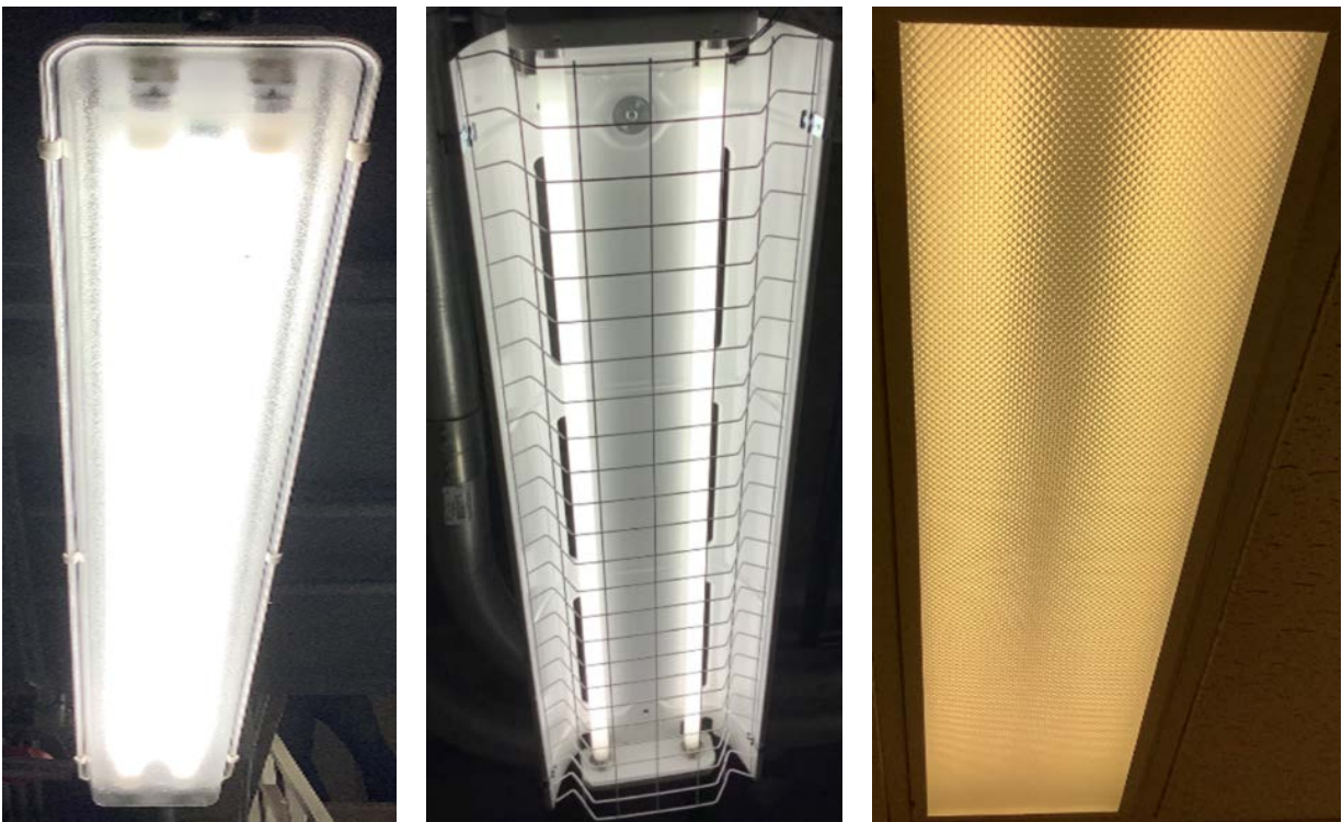
Linear Fluorescent T8 Fixtures
