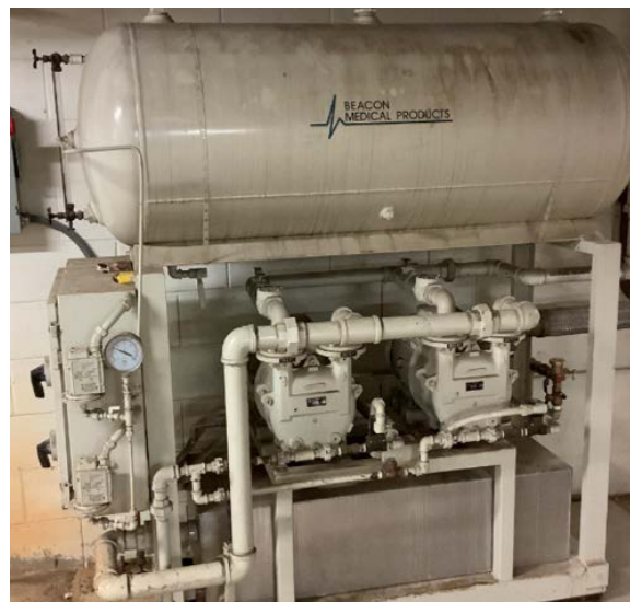
Honeywell & Medical Vacuum Compressors
