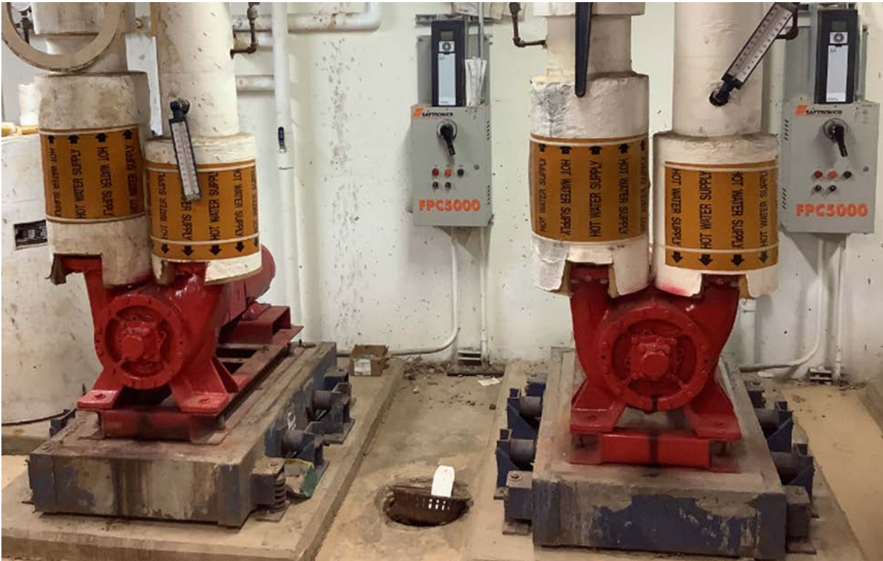
Hot Water Pumps & VFDs - CPM Building
