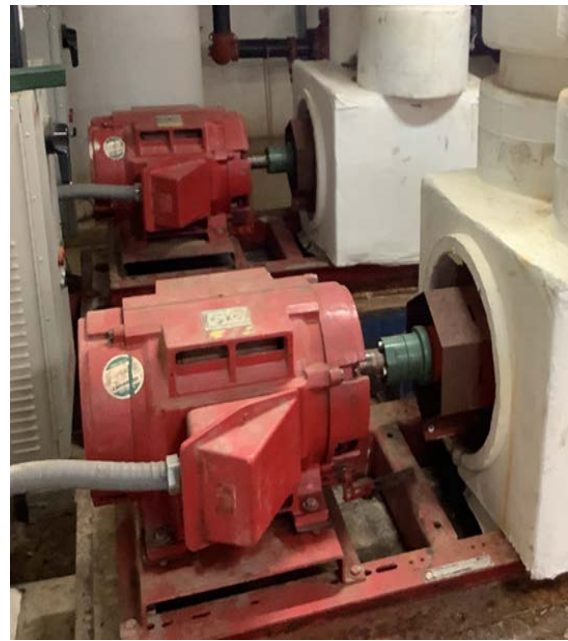
Chilled Water Pumps - CA & CPM Buildings
