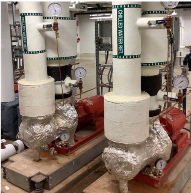
Chilled Water Pumps - CA & CPM Buildings
