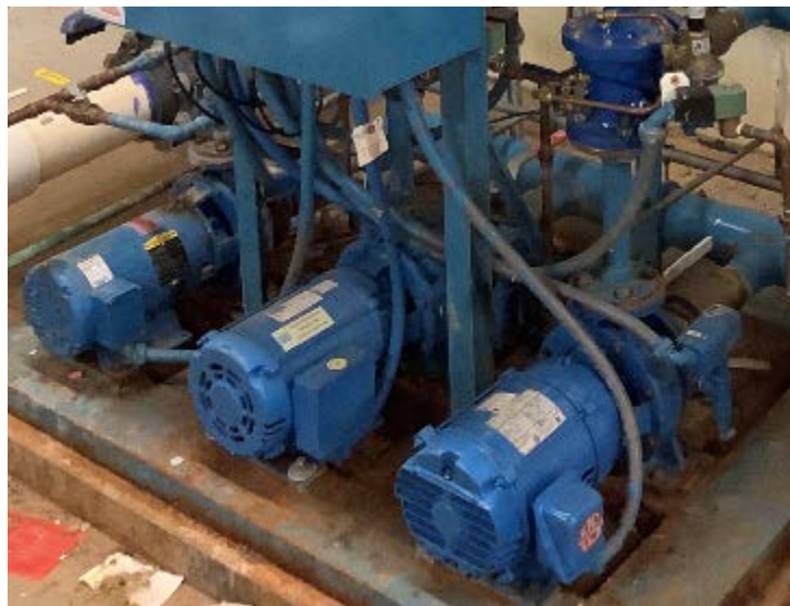
Domestic Cold Water Booster Pumps
