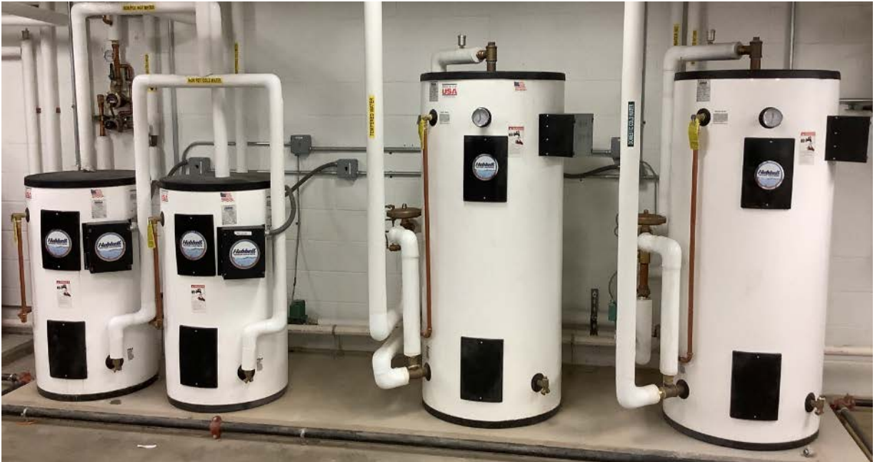
Electric Storage Tank Water Heaters
