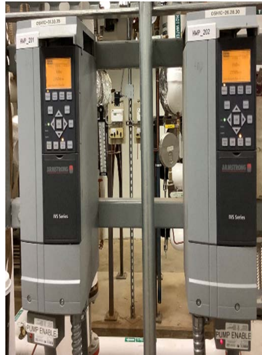
Hot Water Pumps & VFDs - CA Building
