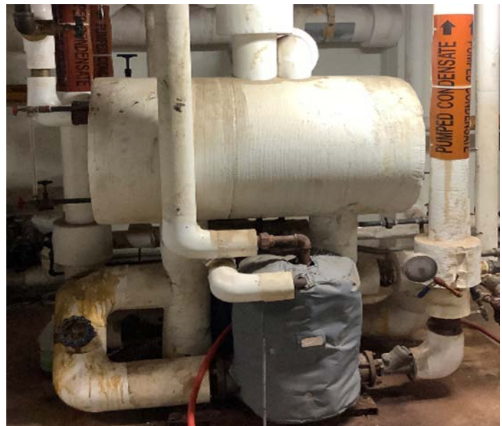
Induce Pressure Condensate Pumps
