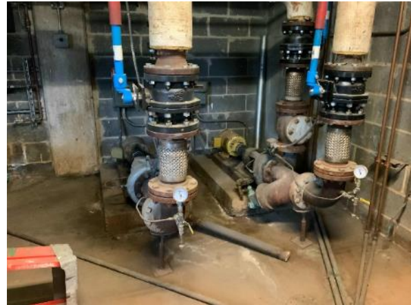
Heating Hot Water Pumps
