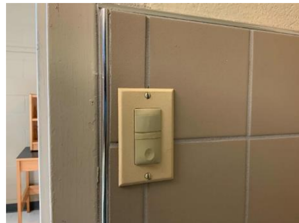
Wall Mounted Occupancy Sensor
