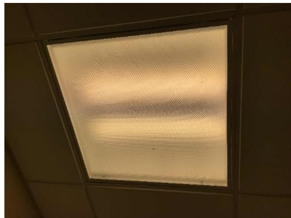
Linear Fluorescent T8 fixtures
