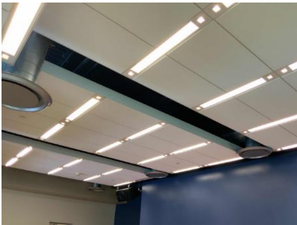
Linear Fluorescent T5 Fixtures
