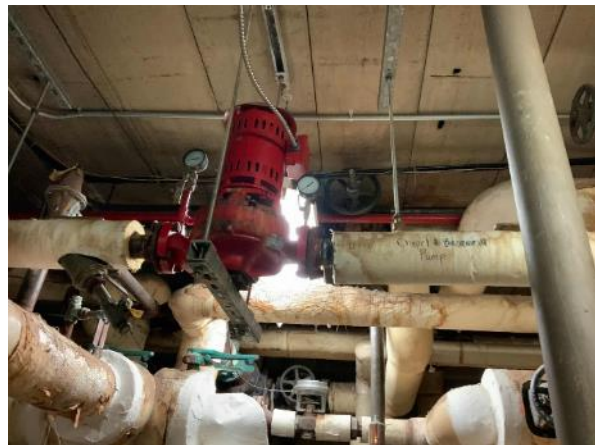
Heating Hot Water Pump serving Chapel
