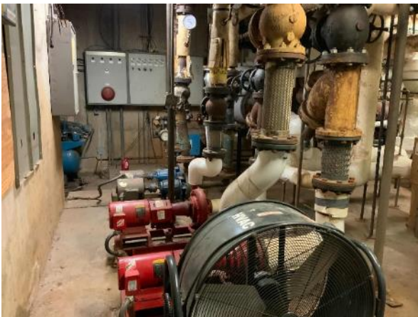
Heating Hot Water Pumps serving Decker
