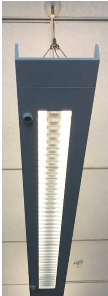
Linear Fluorescent T8 Fixtures
