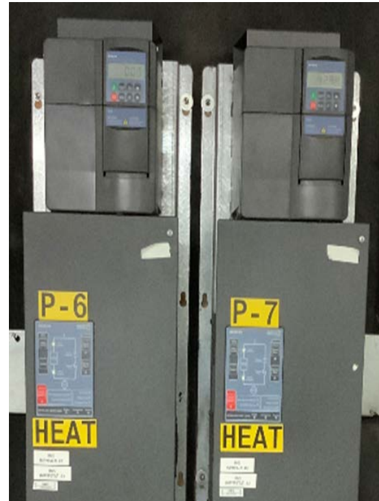
15 hp Pumps & Variable Speed Drives
