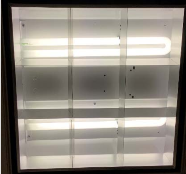
Biaxial CFL Fixtures
