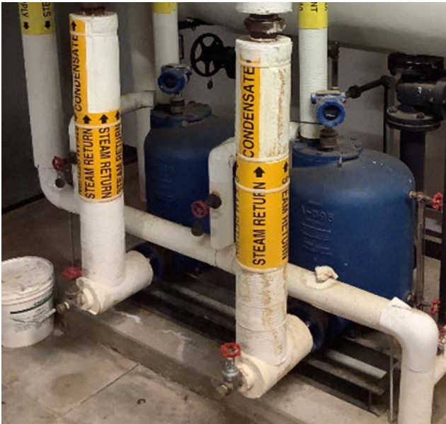
Condensate Pumps & Heat Exchanger
