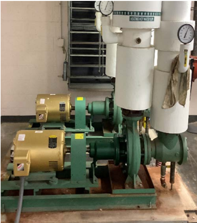
15 hp Pumps & Variable Speed Drives
