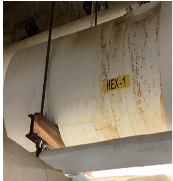
Condensate Pumps & Heat Exchanger
