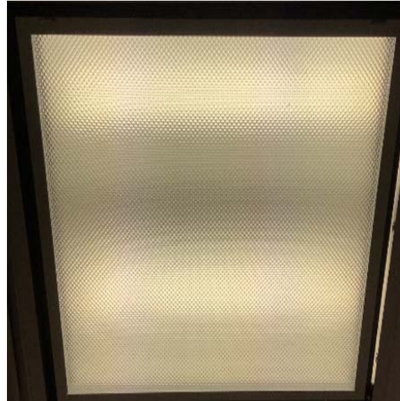
Biaxial CFL Fixtures
