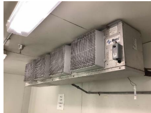
C-Store Walk-In Refrigerator Evaporator
