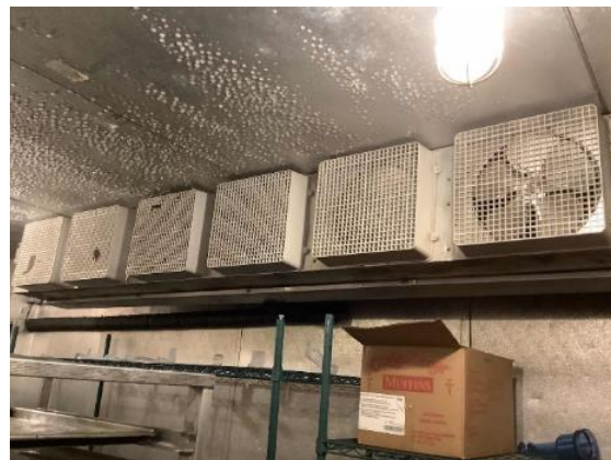
Walk-In Freezer Evaporator Fans
