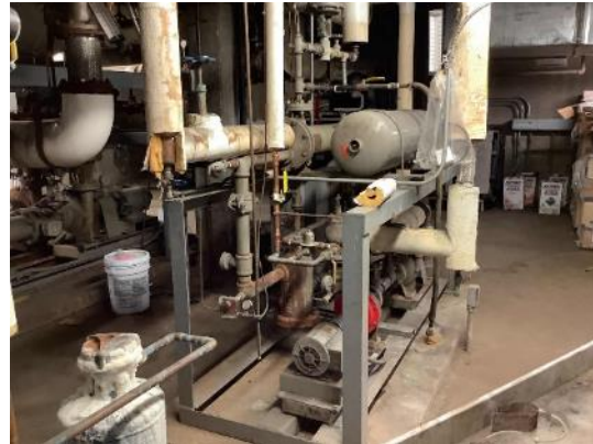
Heat Exchanger for Baseboard Perimeter Heating
