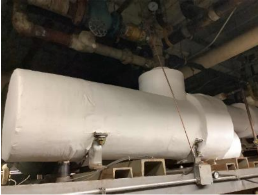
Heat Exchanger for AHUs and HRUs
