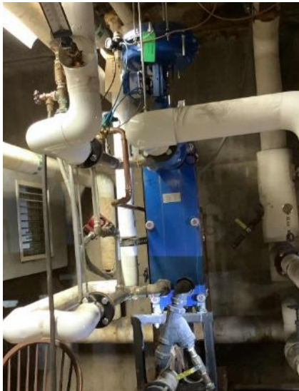
DHW Heat Exchanger
