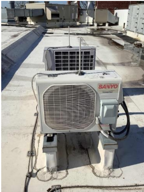
Sanyo Ductless Mini-Split System ACs
