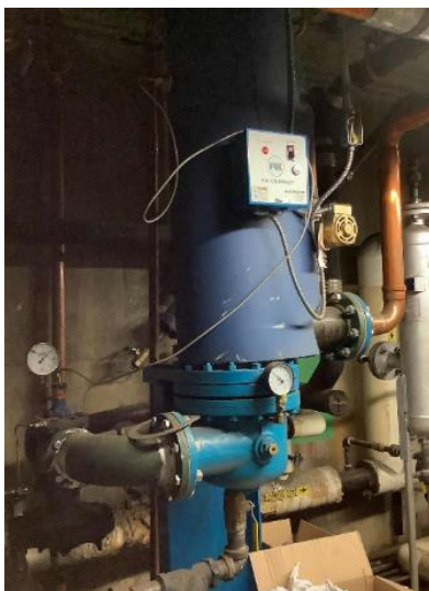
DHW Heat Exchanger
