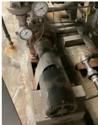
Heating Hot Water Pump
