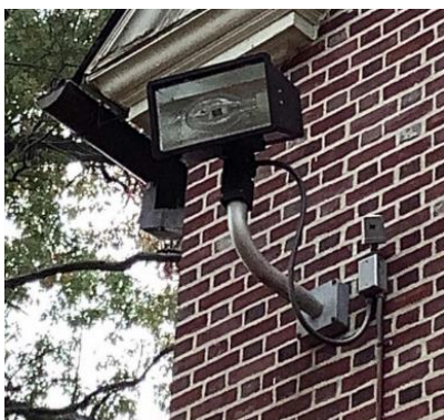
Arm-Mounted Fixture
