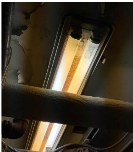
Kitchenette Linear Fluorescent T12 Fixture
