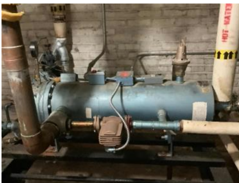
DHW Heat Exchanger
