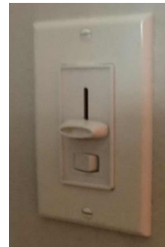
Dimming Switch
