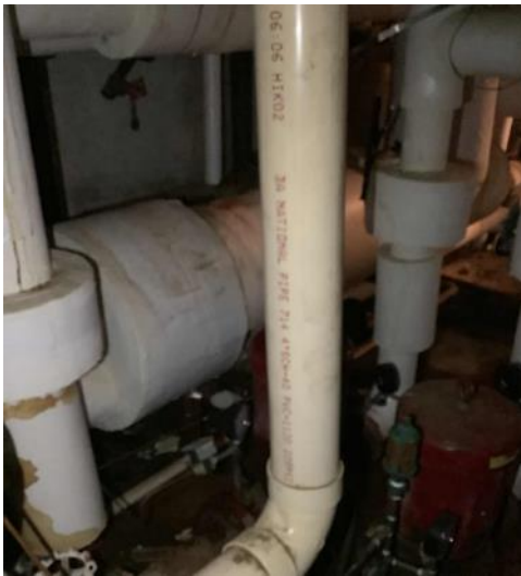
Heating Heat Exchanger
