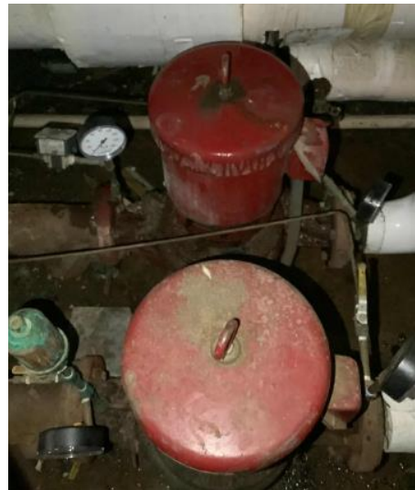
Heating Hot Water Pumps
