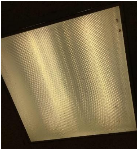
Hallway Linear Fluorescent T8 Fixture
