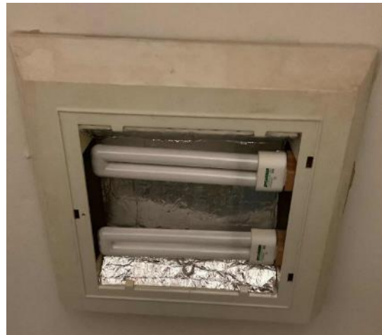
Janitorial Closet CFL Ceiling Mounted Fixture
