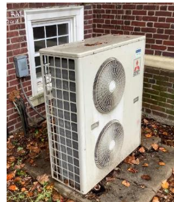
Ductless Mini-Split System AC
