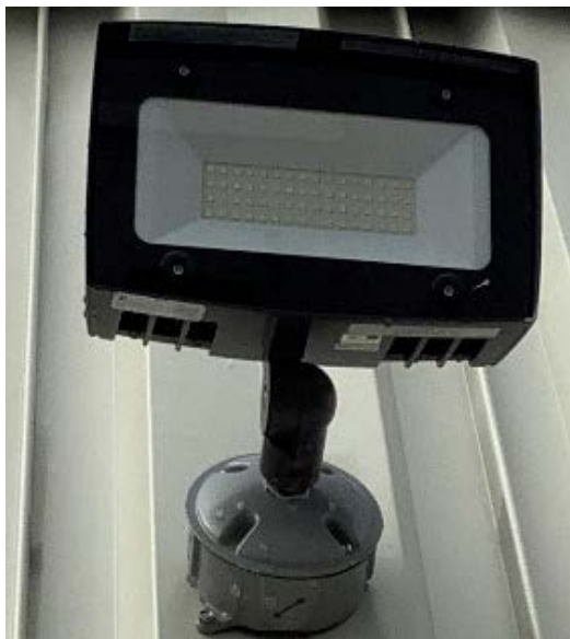
The Roof LED Fixture & Timeclock
