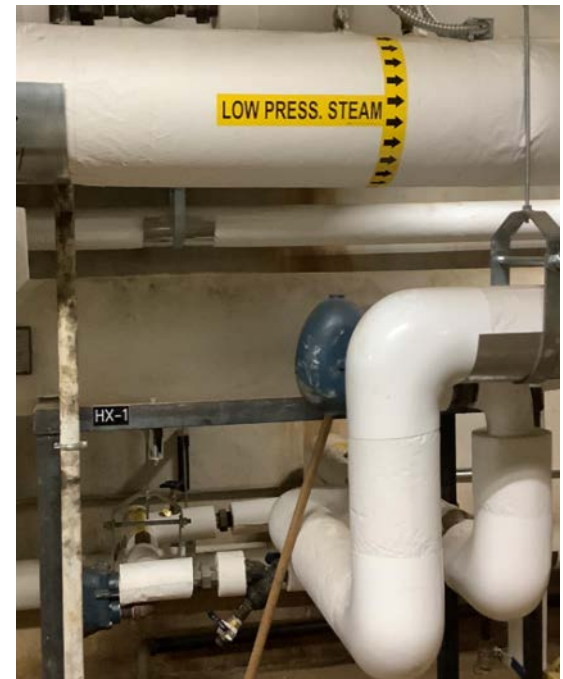
Condensate Pumps & Heat Exchanger
