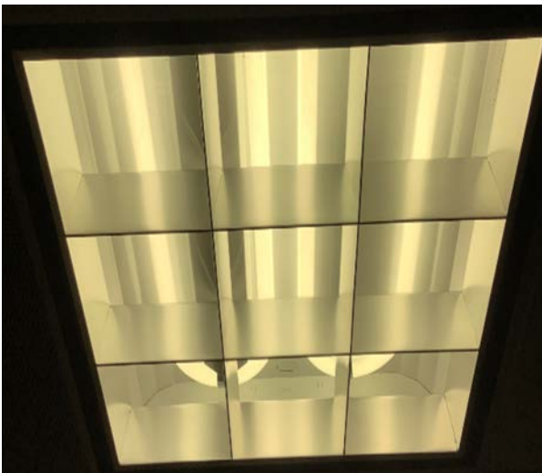
U-Bend T8 & Biaxial CFL Fixtures
