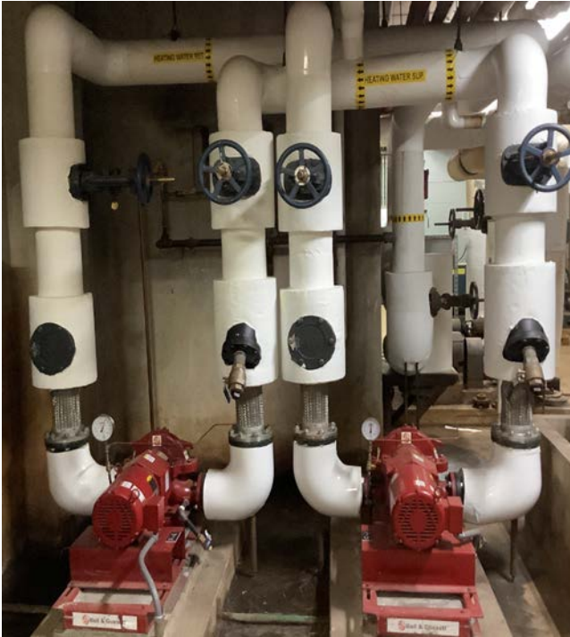
10 hp Hot Water Distribution Pumps % Variable Frequency Drives (VFDs)
