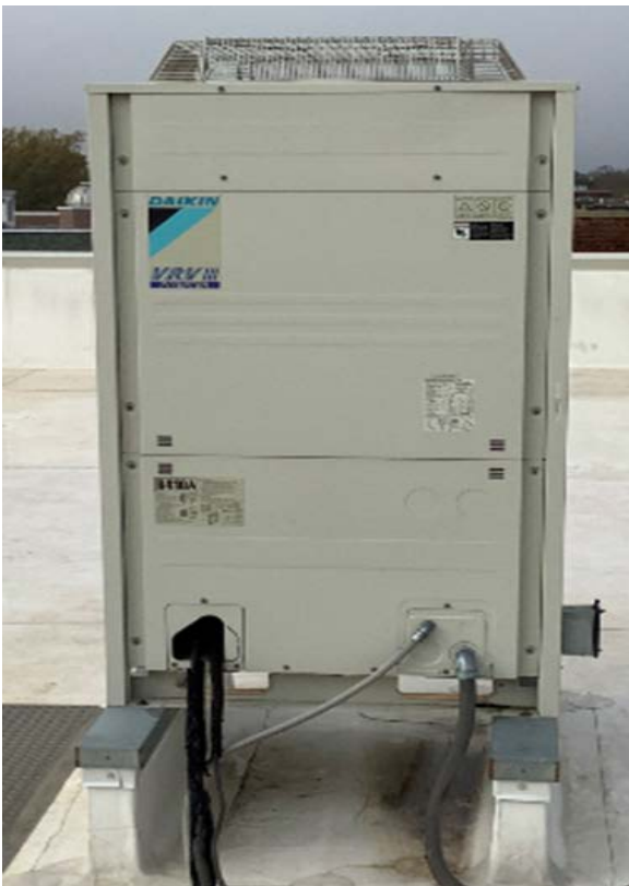
6-Tons Daikin Split Heat Pump & Programmable Thermostat
