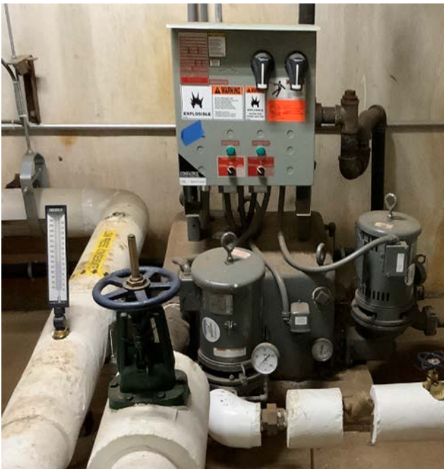
Condensate Pumps & Heat Exchanger
