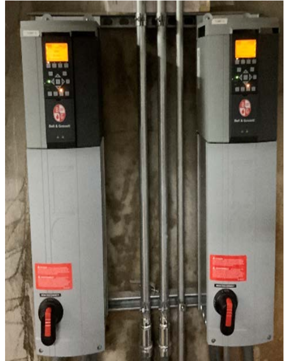
10 hp Hot Water Distribution Pumps % Variable Frequency Drives (VFDs)
