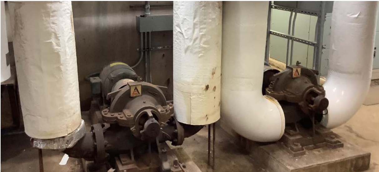
25 hp Chilled Water Pumps
