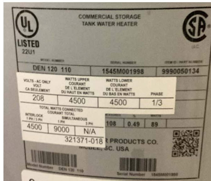
120 Gallon Electric Storage Tank Water Heater
