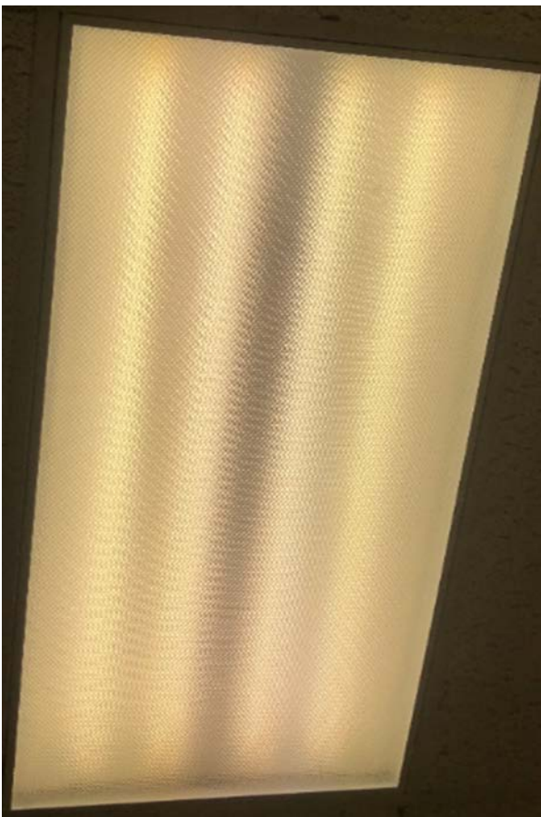
Linear Fluorescent T8 Fixtures
