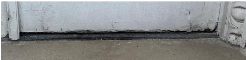
Damage Door Seal
