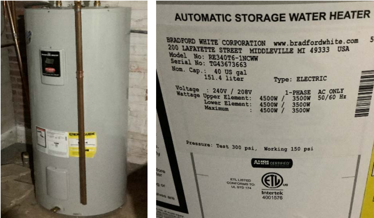
Electric Storage Tank Water Heater
