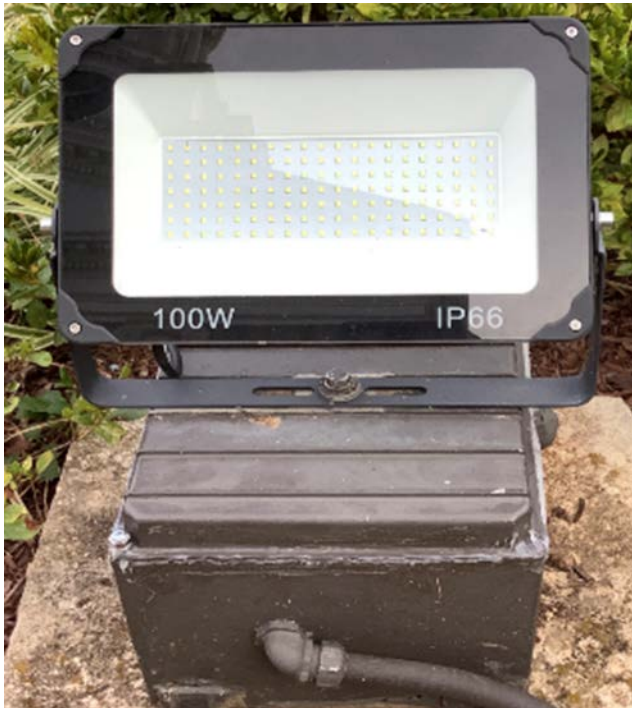
LED Landscape Spot Luminaire & CFL Fixture
