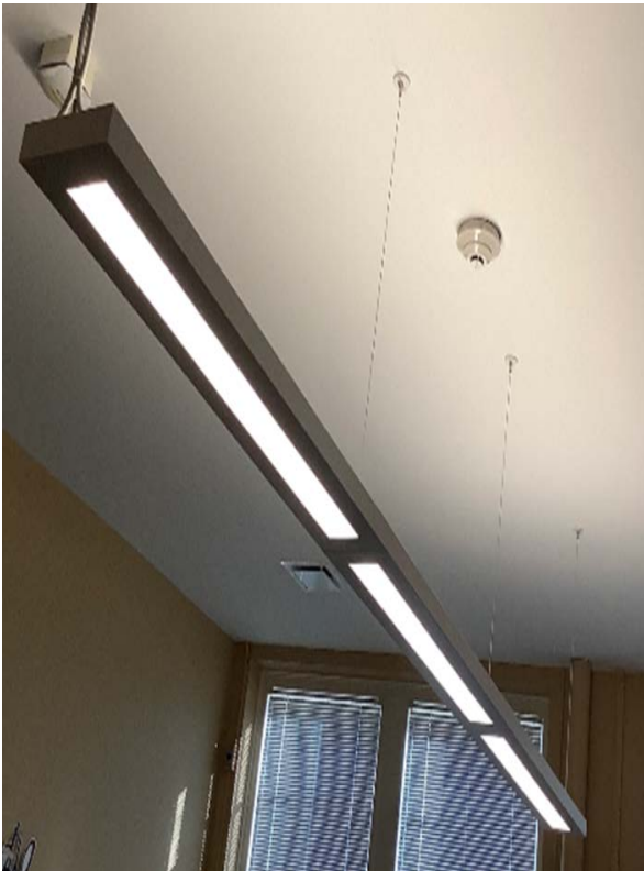
Pendant LED Fixtures & LED Exit Signs
