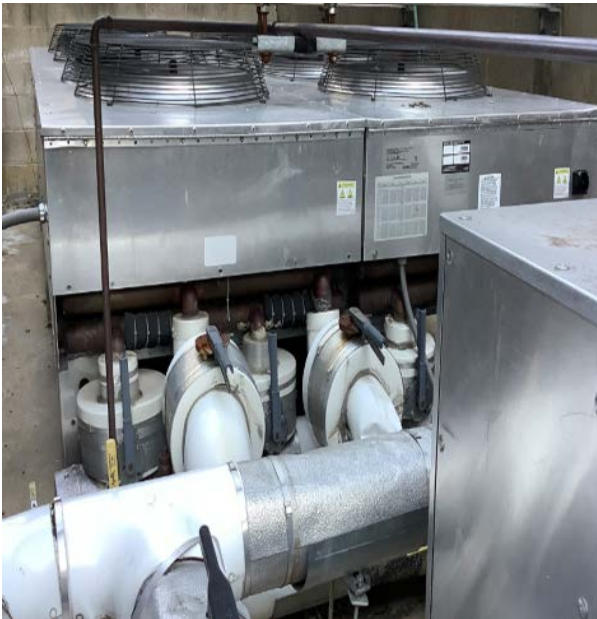
Liebert Outdoor Condensing Units & Digital Control Panel
