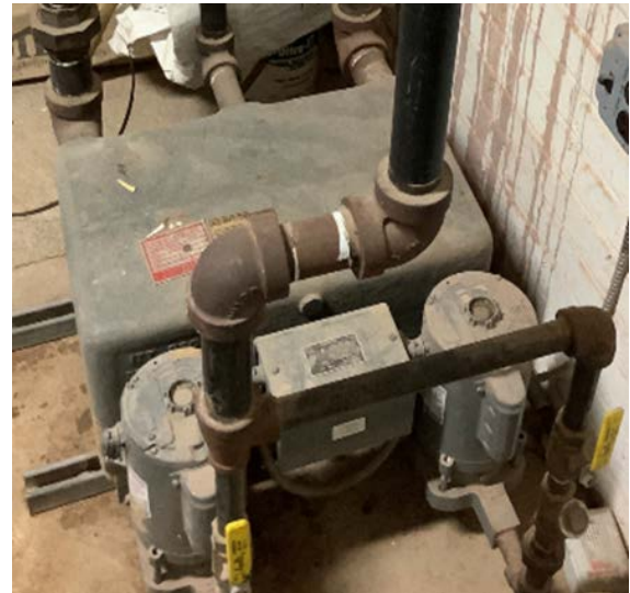
Heat Exchanger & Condensate Pumps
