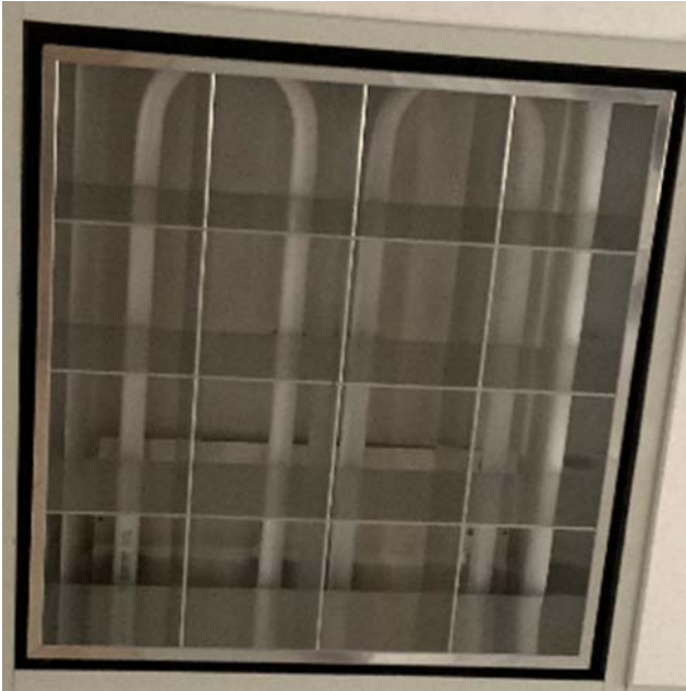
U-Bend Tubes & LED Lamps
