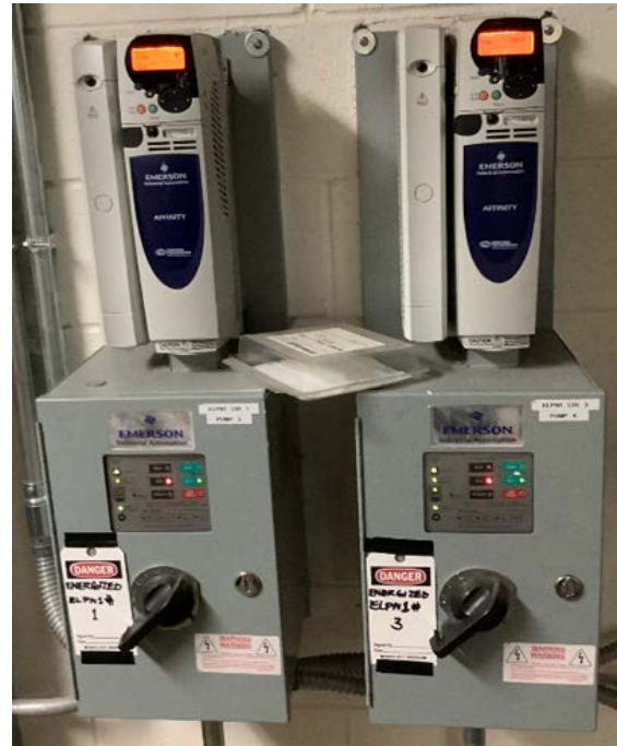
Hot/CHW Recirculation Pumps & VFDs
