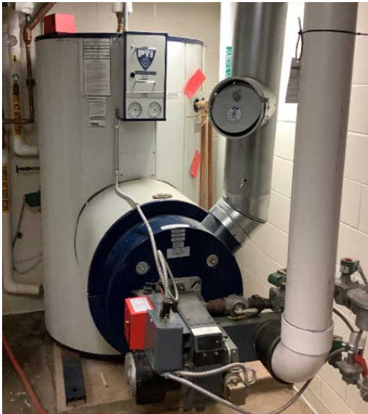
Gas-Fired Water Heater, Pipes & Pumps
