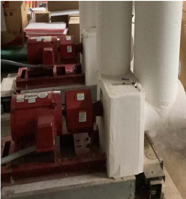
Hot/CHW Recirculation Pumps & VFDs
