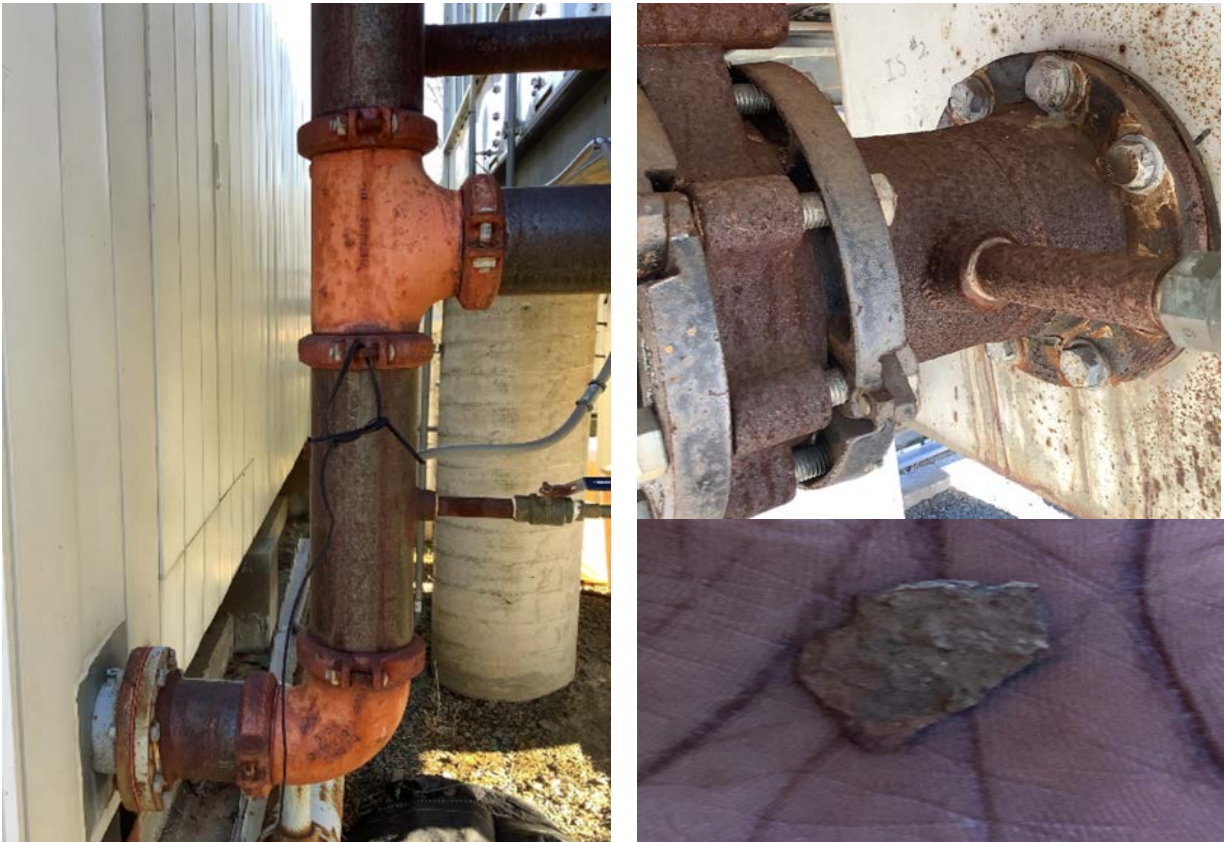
Corroded Metal Pipes
