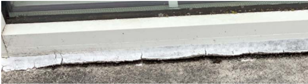
Exterior Doors & Signs of Damaged Fiberglass Thermal Break
