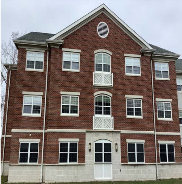
Brick Veneer & Concrete Unit Walls
