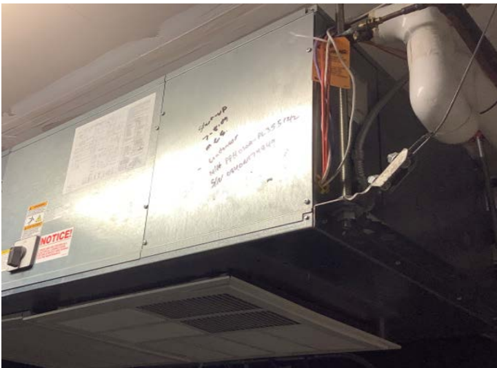
Indoor Evaporator & Programmable Thermostat
