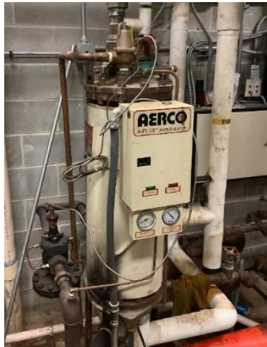
DHW Heat Exchanger
