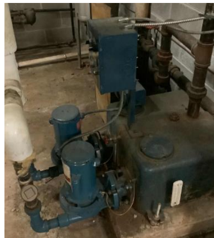
Heating Hot Water Condensate Pumps
