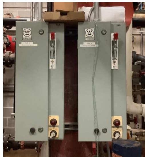
Chilled Water Pump Controls
