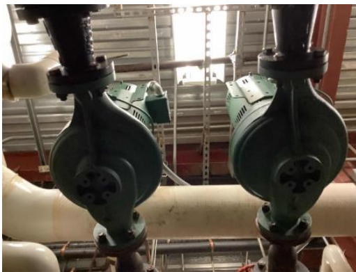
Heating Hot Water Pumps
