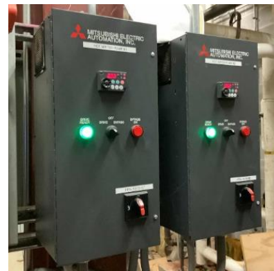
Heating Hot Water Pump Controls
