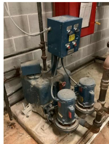
DHW Condensate Pumps
