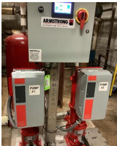
Domestic Water Pressure Pumps
