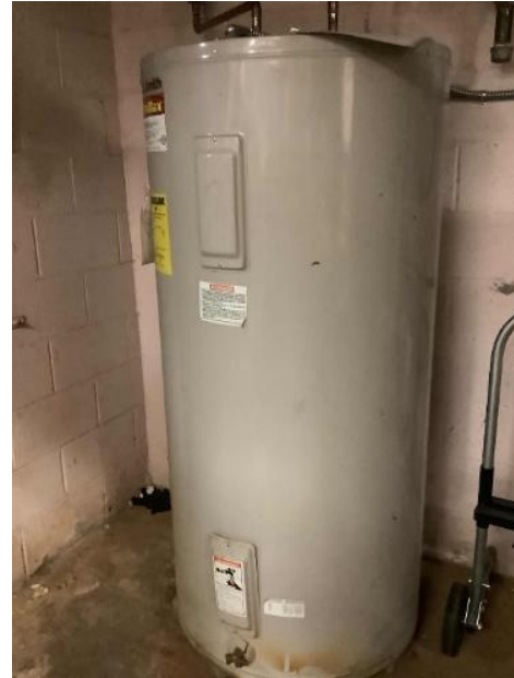
Electric DHW Storage Tank Water Heater
