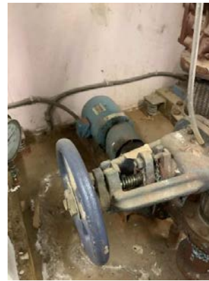
Heating Hot Water Pump
