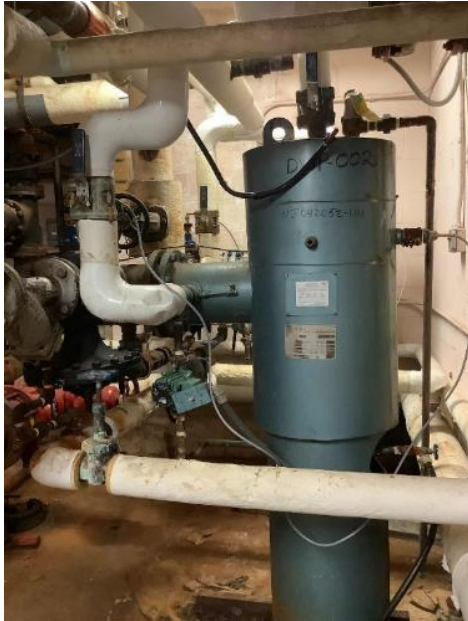
DHW Heat Exchanger
