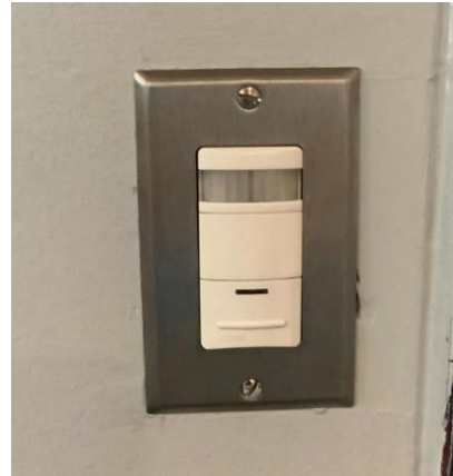
Wall Mounted Occupancy Sensor
