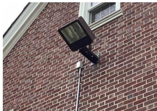
Metal Halide Arm Mounted Fixture
