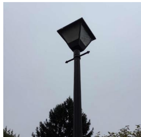
LED Pole Mounted Fixture
