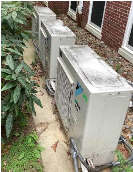
Ductless Mini-Split System AC Units
