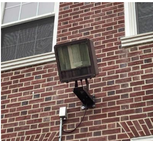
LED Arm Mounted Fixture
