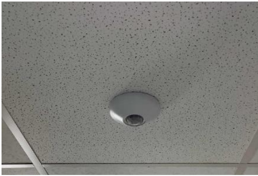
Ceiling Mounted Occupancy Sensor
