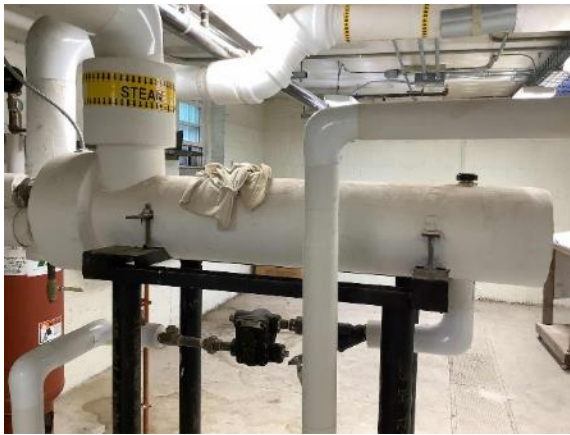
Heating Heat Exchanger
