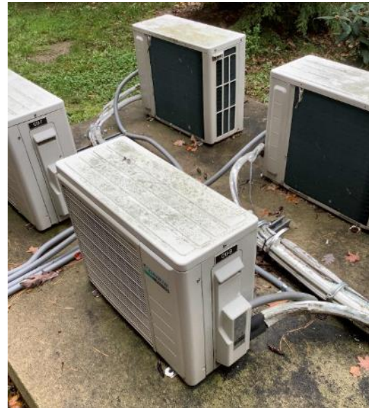
Ductless Mini-Split System AC Units
