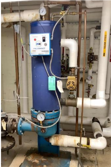
DHW Heat Exchanger
