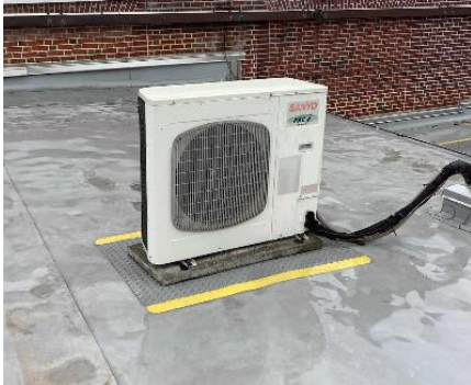
Ductless Mini-Split System AC
