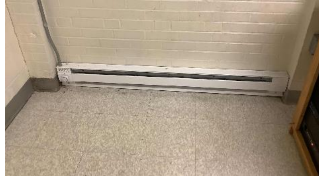
Electric Resistance Baseboard Heater
