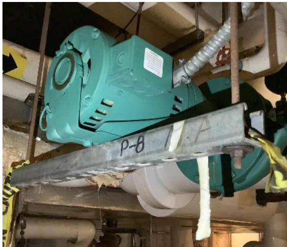
Heating Hot Water Pump 8
