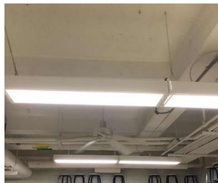
Locker Room Pendant Mounted Fixtures
