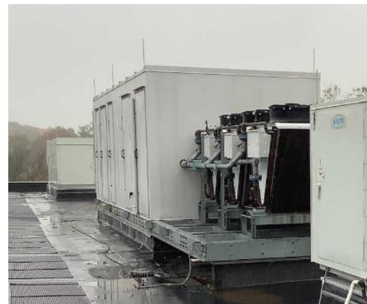
AHU-1 Pool Room Dehumidification Unit
