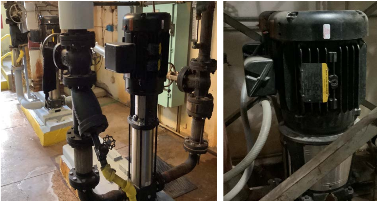
Boiler Plant & Cogeneration Plant Feedwater Pumps
