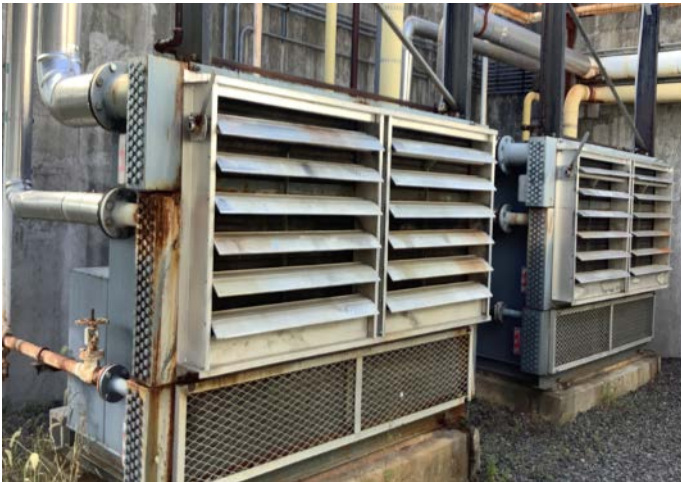
High Pressure Gas Coolers
