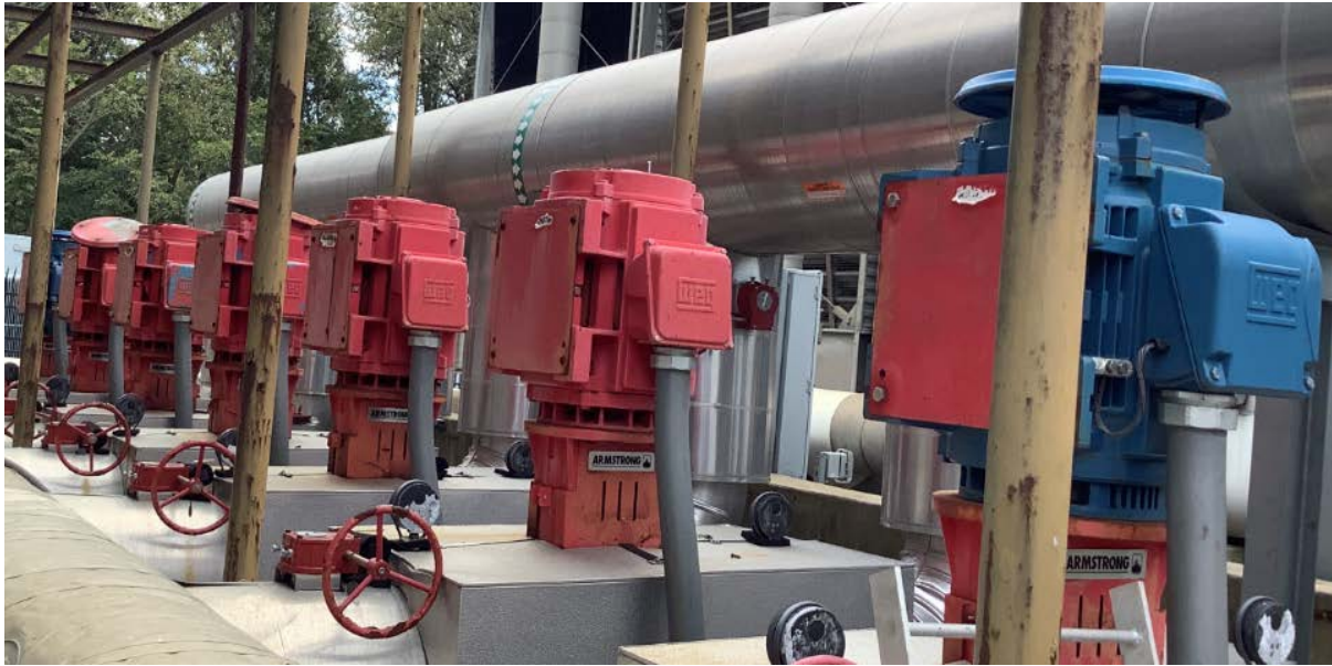
Condenser Water Pumps
