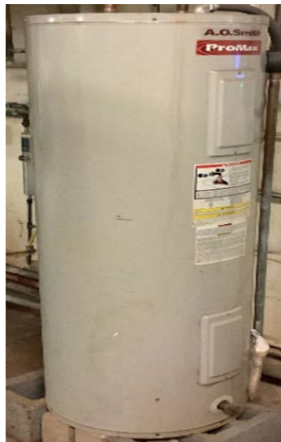
40 Gallon Electric Water Heater
