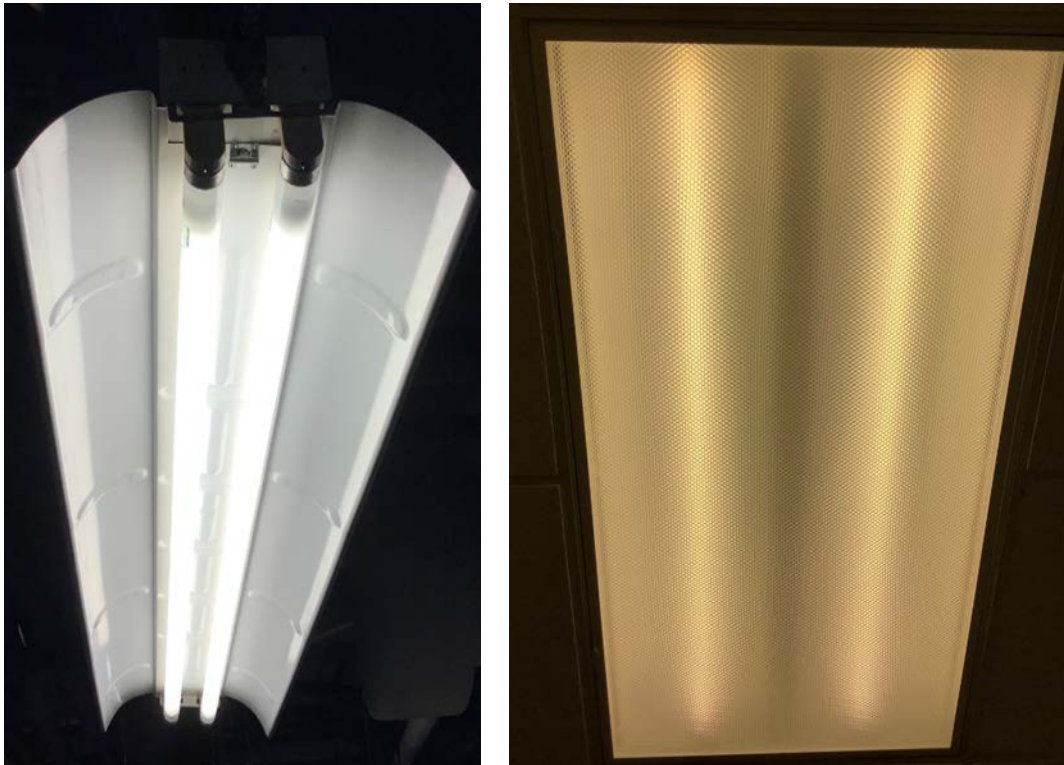
Linear Fluorescent T8 Fixtures
