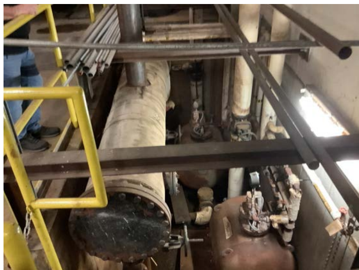
High Pressure Condensate Return Flash Tank
