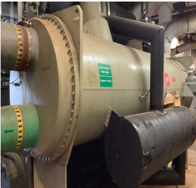
Trane Centrifugal Chiller #5
