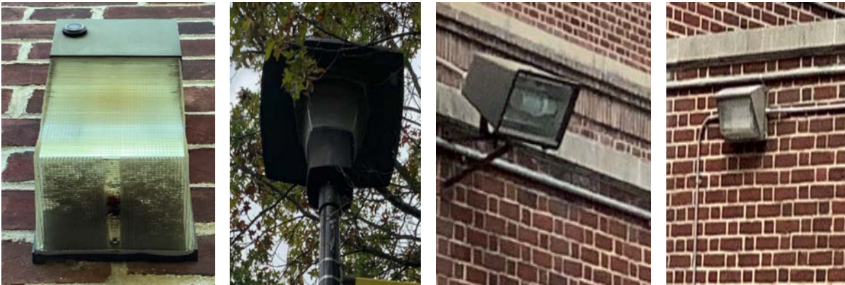
CFL & LED Exterior Fixtures
