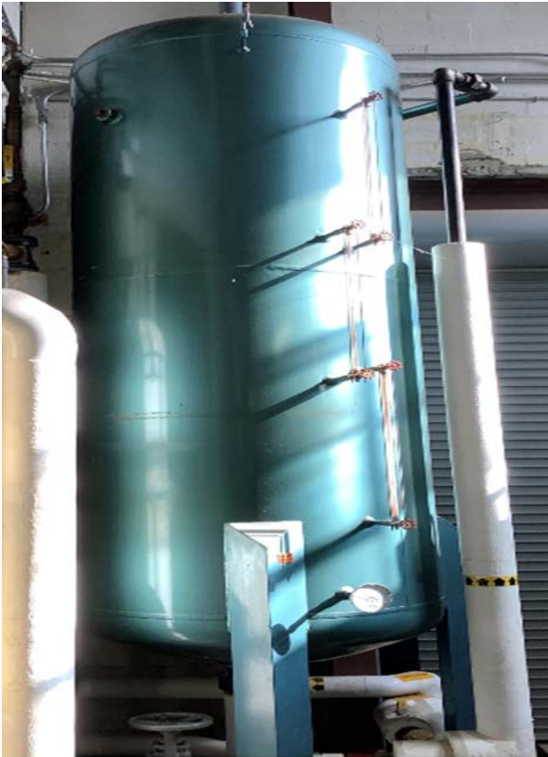
Boiler Blowdown Tank
