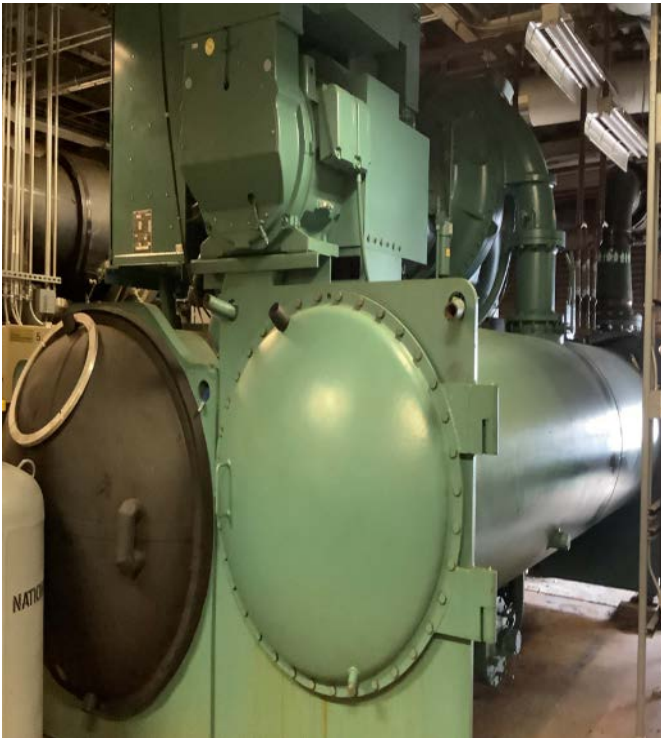
Electric Chiller #3 with Variable Speed Drive
