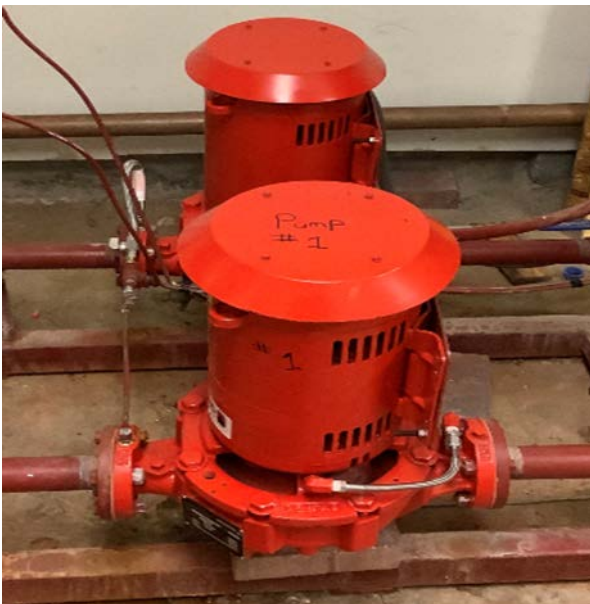
Domestic Cold Water Booster Pumps (P1P2)
