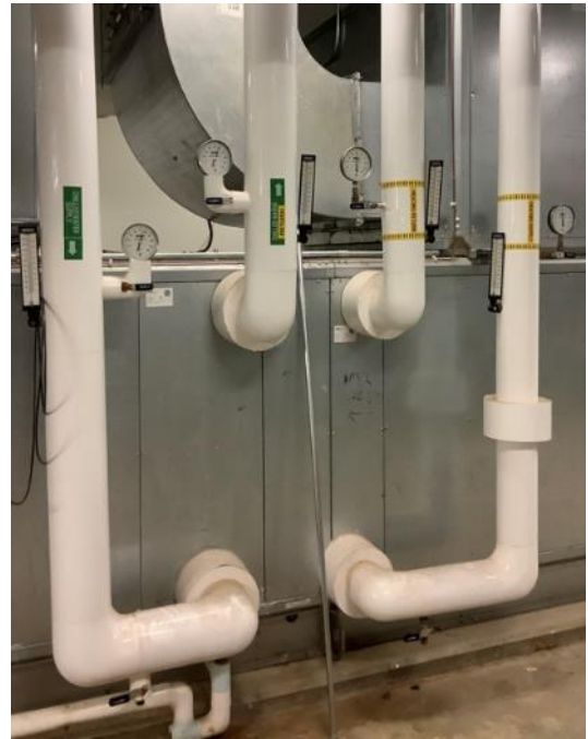
AHU-5, Hot Water & Chilled Water Pipes
