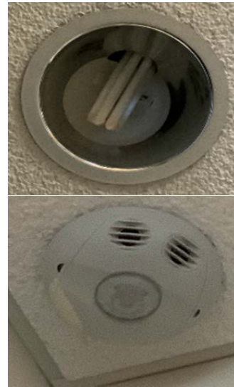
Honeywell Controller, CFL Recessed Can & Ceiling Mounted Occupancy Sensor
