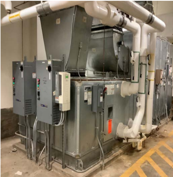
AHU-5, Hot Water & Chilled Water Pipes
