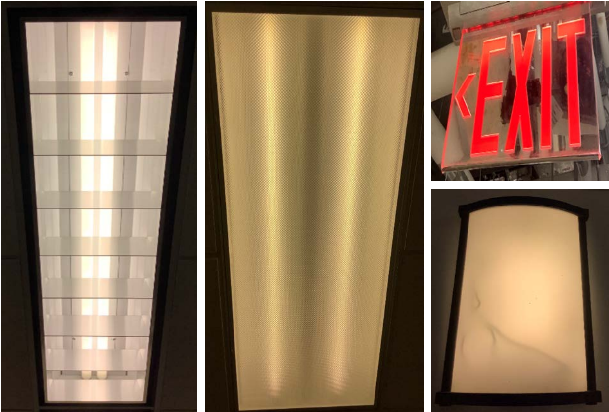
T8 Recessed Fixtures, LED Exit Sign & Wall Mounted CFL Lamp
