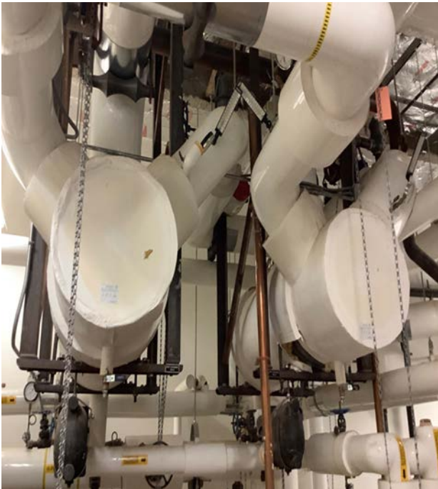
Heat Exchangers & Condensate Pumps
