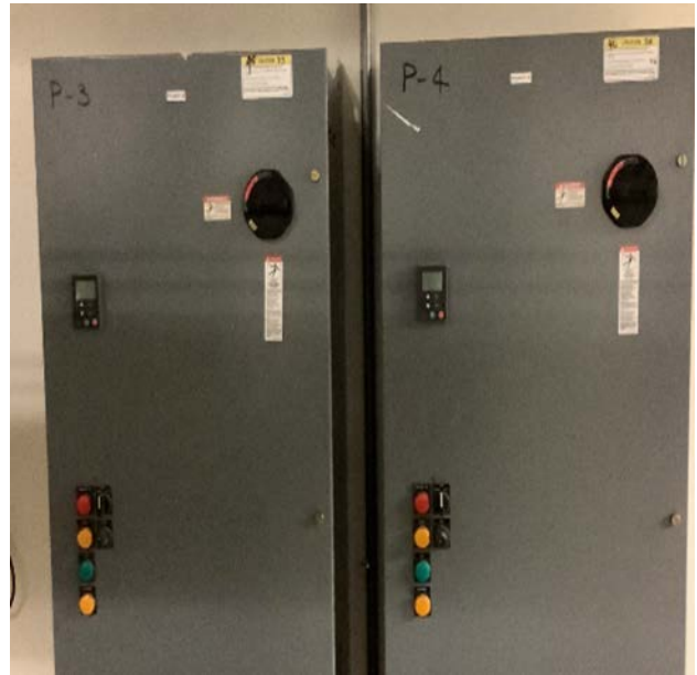
Chilled Water Pumps (CHP3,4) & Variable Speed Drives (VFDs)
