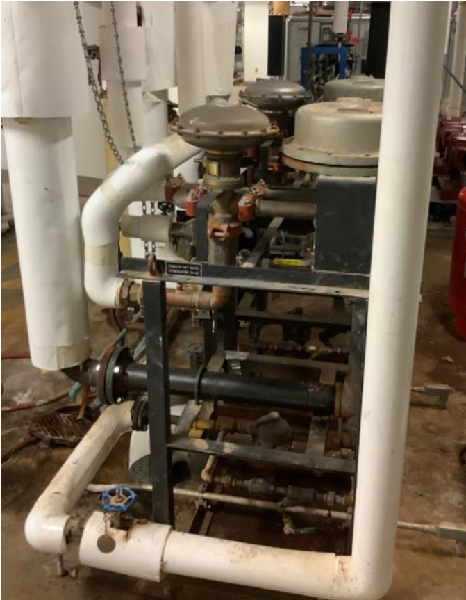
Domestic Hot Water Generator Through Heat Exchanger
