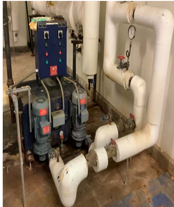
Heat Exchangers & Condensate Pumps
