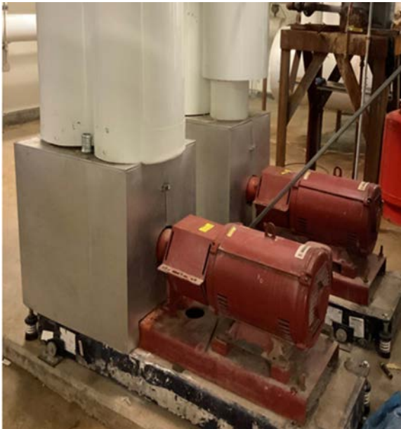
Chilled Water Pumps (CHP3,4) & Variable Speed Drives (VFDs)
