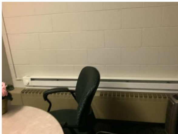
Electric Resistance Heater
