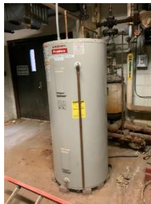
Electric Storage Tank Water Heater
