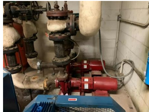
Heating Hot Water Pumps
