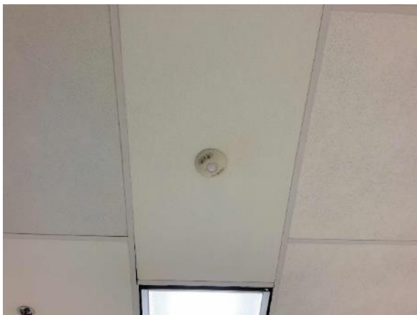
Ceiling Mounted Occupancy Sensor
