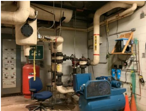
Steam Heat Exchanger
