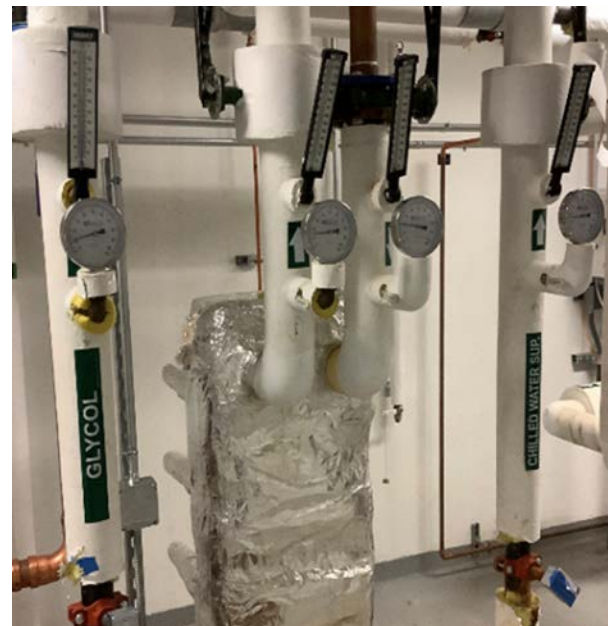
7.5 hp Process Cooling Water Pumps & Heat Exchanger
