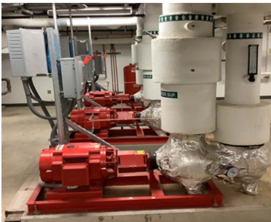
Chilled Water Pumps & Variable Frequency Drive (VFD)
