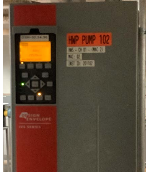
Hot Water Pumps & Variable Frequency Drive (VFD)
