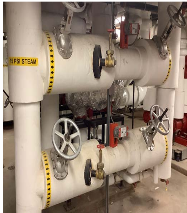
Pressure Induce Condensate Pumps & Heat Exchangers
