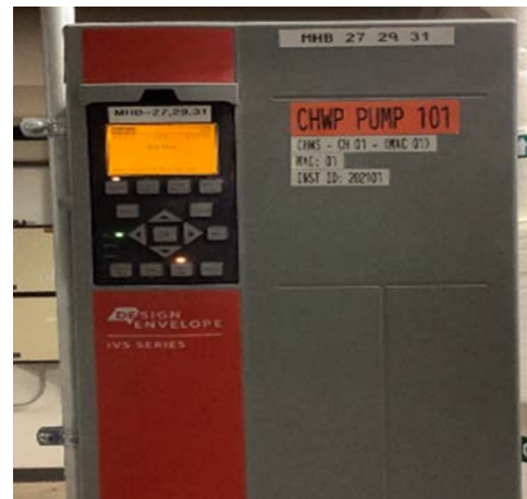
Chilled Water Pumps & Variable Frequency Drive (VFD)
