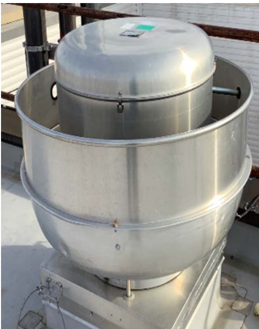
Exhaust Fan 107 (3 hp) & Variable Frequency Drives (VFDs)
