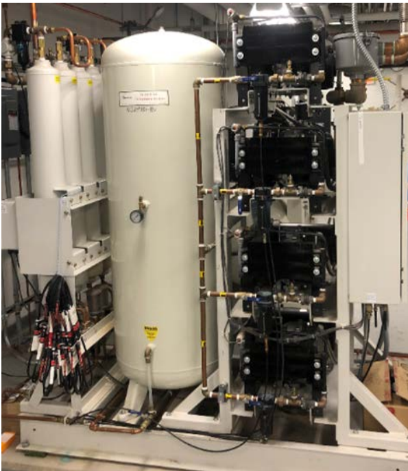
Four 5 hp & Two 15 hp Compressors
