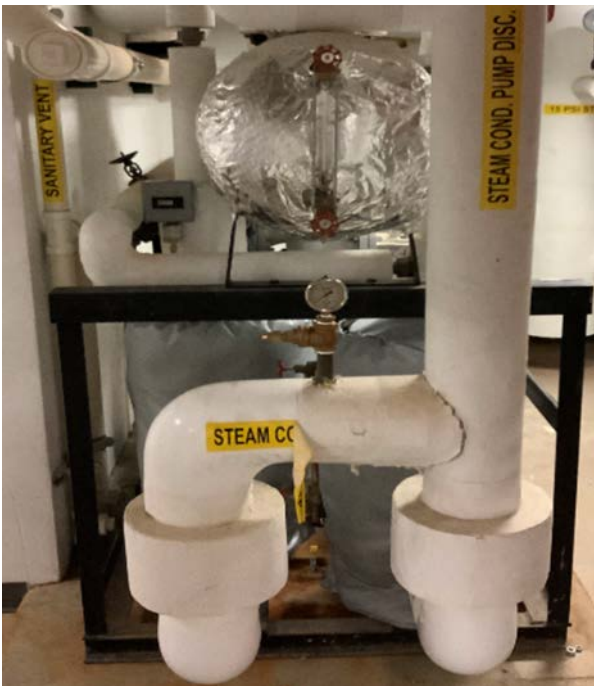
Pressure Induce Condensate Pumps & Heat Exchangers
