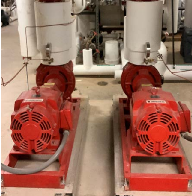
Hot Water Pumps & Variable Frequency Drive (VFD)
