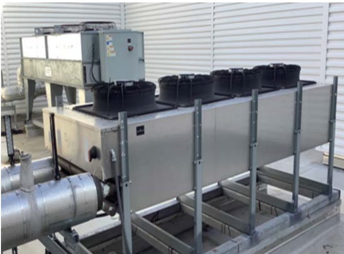
Colmac Fluid Cooler
