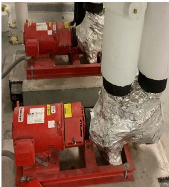
7.5 hp Process Cooling Water Pumps & Heat Exchanger
