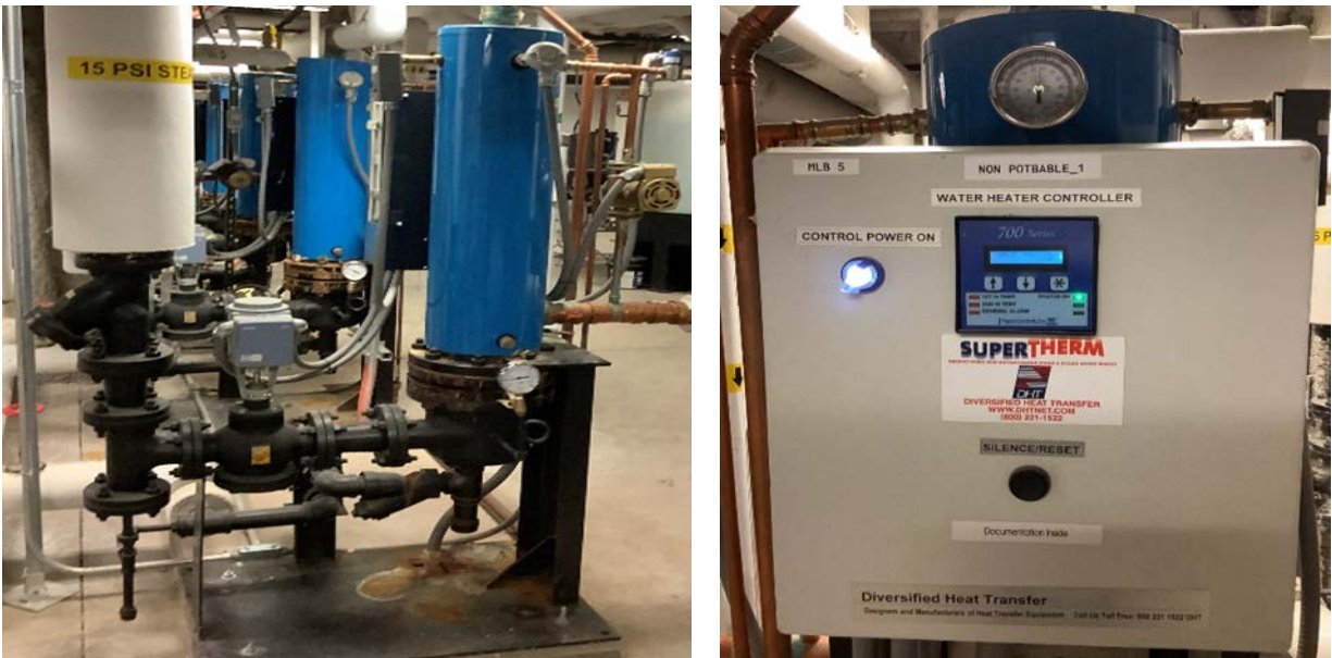
Indirect Fired Semi-Instantaneous Water Heaters & Control Panel
