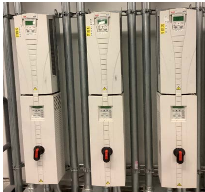
Exhaust Fan 107 (3 hp) & Variable Frequency Drives (VFDs)
