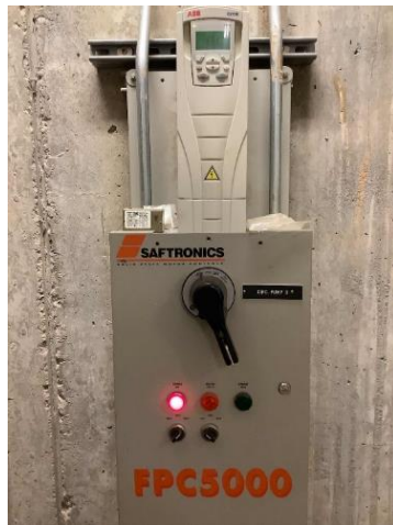
Hot Water Pump Controls
