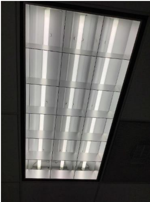
Hallway Linear Fluorescent Fixture
