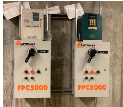
Chilled Water Pump Controls
