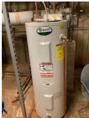
Electric Storage Tank Water Heater
