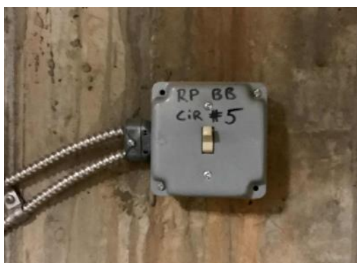
DHW Circulation Pump Control
