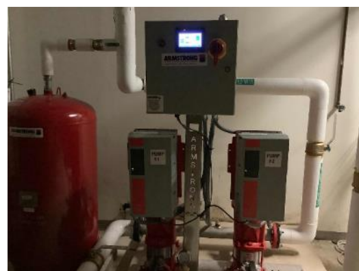
Cold Water Pressure Pumps
