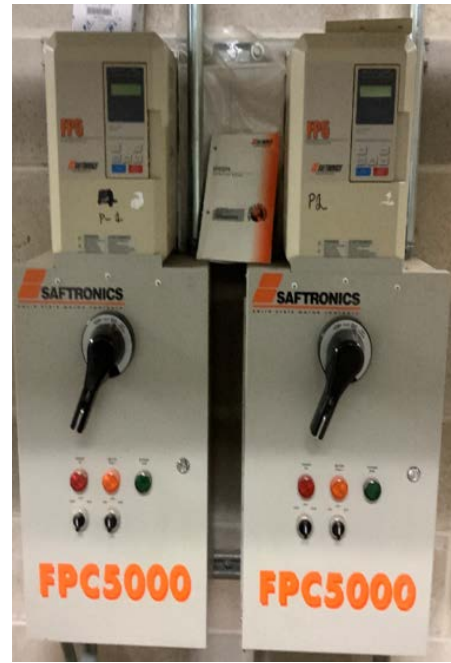
Chilled Water Pumps & Variable Frequency Drives (VFDs)
