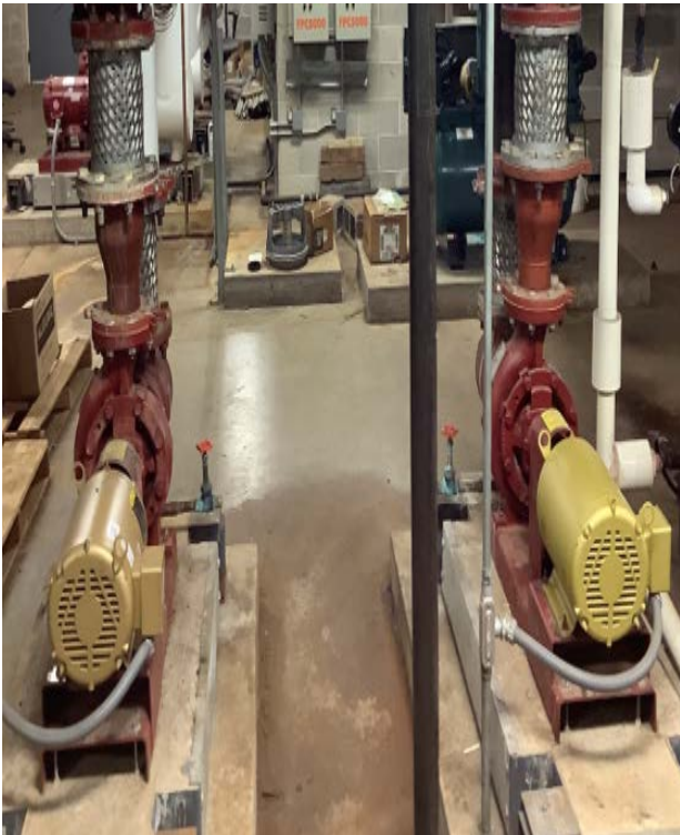
Hot Water Pumps & Variable Frequency Drives (VFDs)
