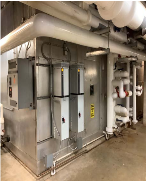
AHU-1, Hot Water & Chilled Water Pipes
