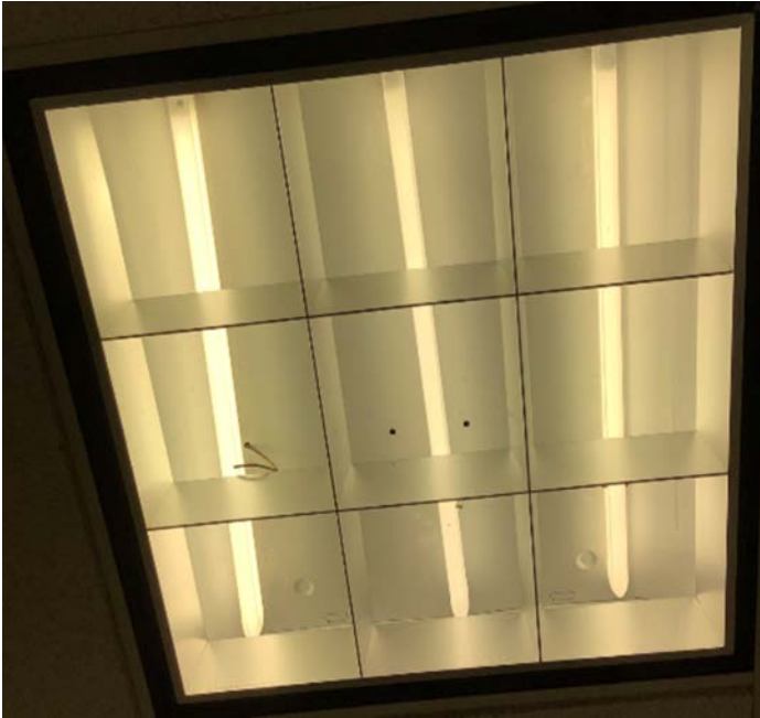
31-Watt Biaxial and 24-Watt CFL Lamps
