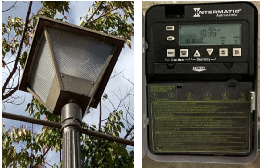
Pole Mounted Walkway LED Fixture & Timeclock
