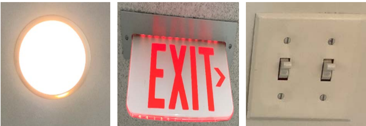
CFL Recessed Can, LED Exit Sign & Wall Switches
