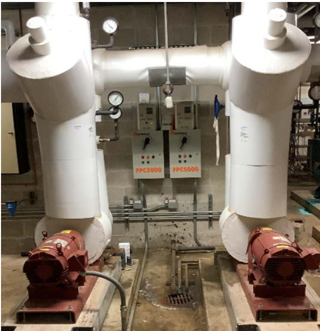
Chilled Water Pumps & Variable Frequency Drives (VFDs)
