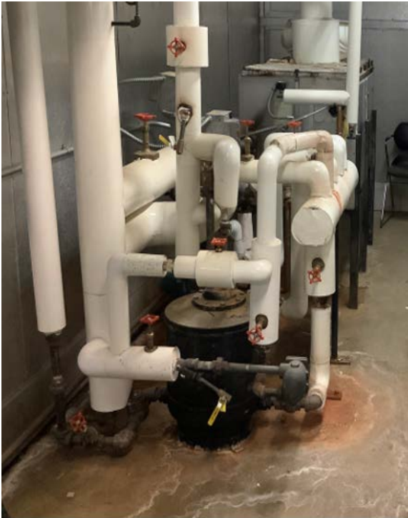
Pressure Induce Condensate Pumps & Steam to Steam Humidifier
