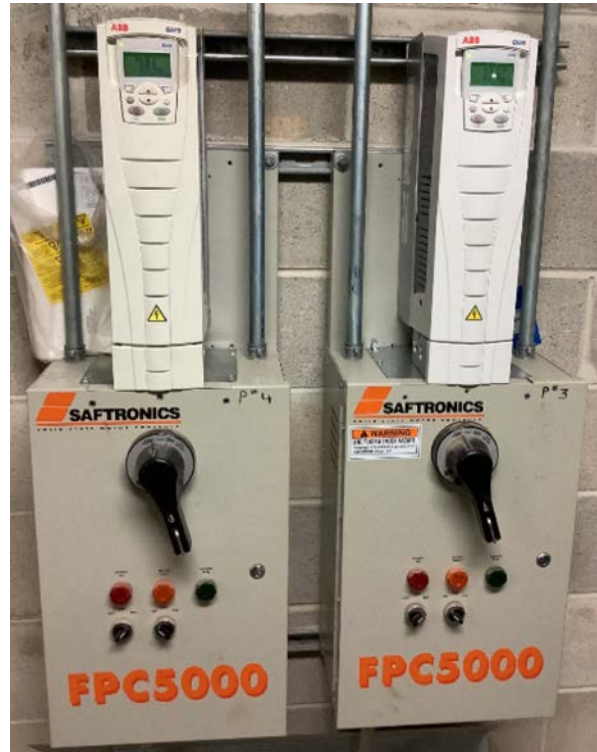
Hot Water Pumps & Variable Frequency Drives (VFDs)
