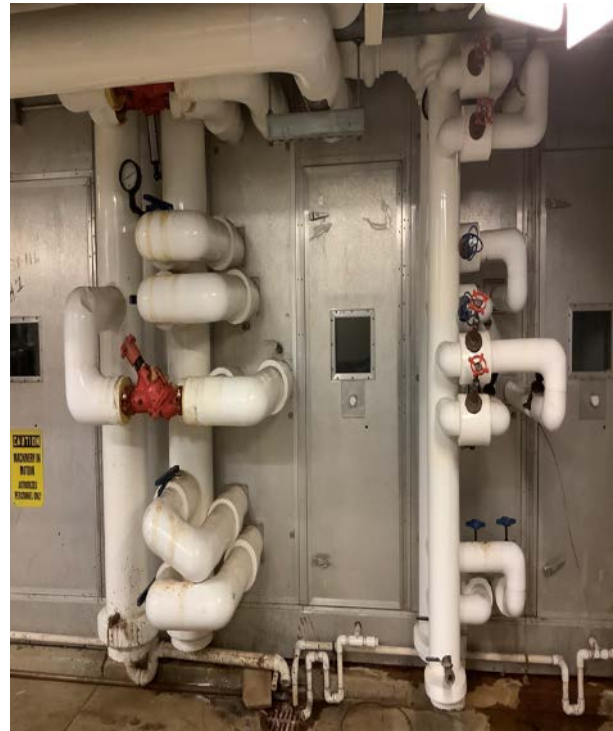
AHU-1, Hot Water & Chilled Water Pipes
